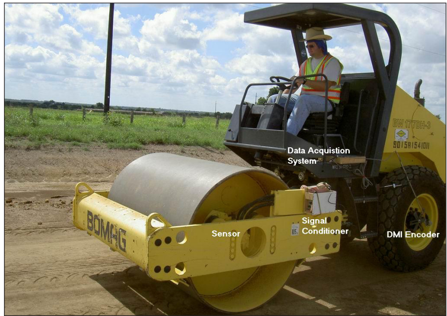
Figure 1. Field-Testing the Instrumented Roller System.
