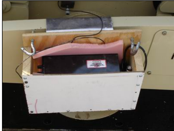
Figure 4. Mounting of Signal Conditioner on Body of Roller.
