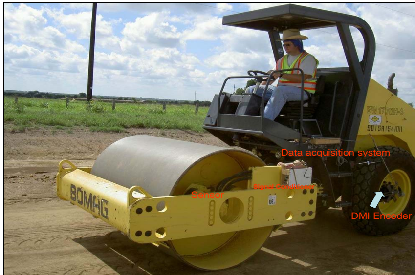
Figure 1. Prototype Compaction System.
