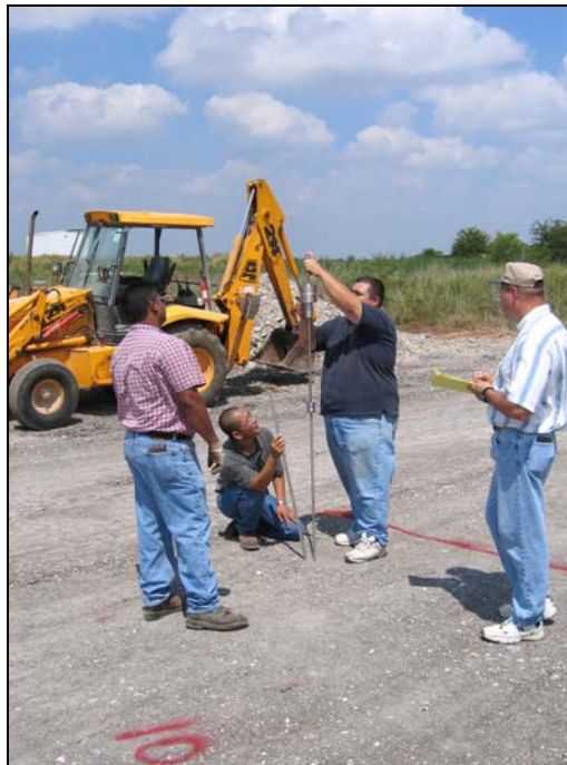
Figure 1.11. Testing with Dynamic Cone Penetrometer.
