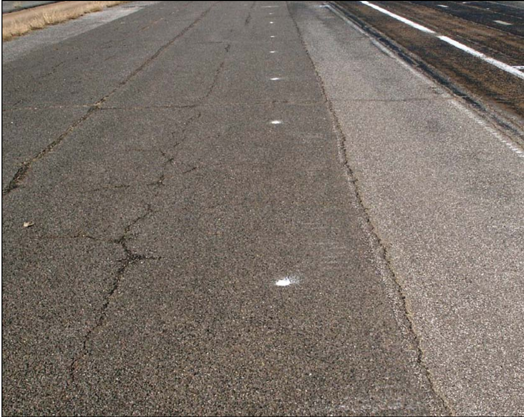
Figure 3.14. Old Seal Coat Pavement Used for Profile Measurements.
