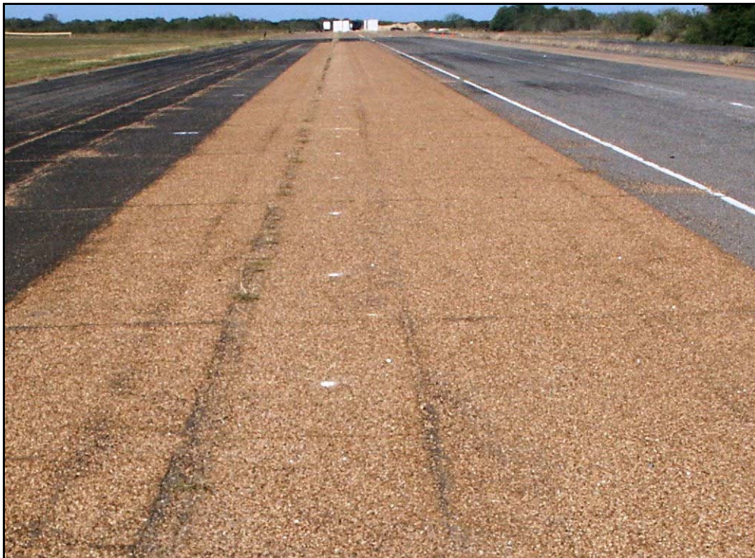
Figure 4.10. Left Seal Coat Section Used for Laser Testing.
