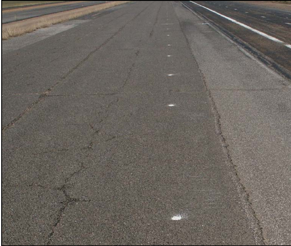
Figure 4.11. Middle Seal Coat Section Used for Laser Testing.
