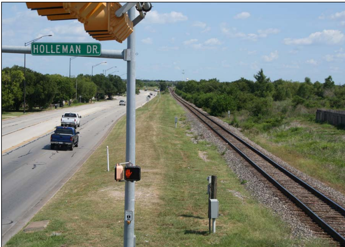
Figure 30. Holleman Drive Intersection.
