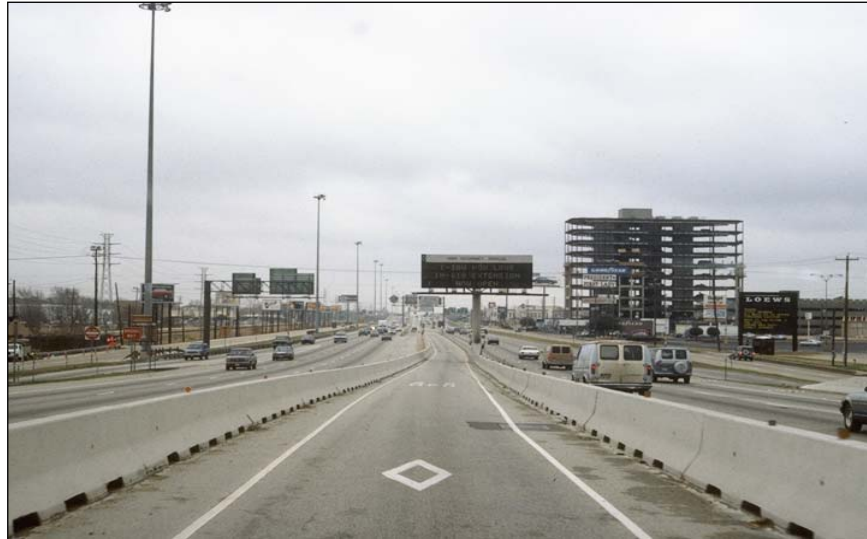
Figure 2. Houston Barrier-Separated HOV Lane Cross Section.
