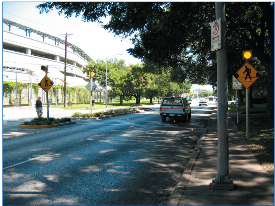
Figure 1. In-Roadway Warning Lights in Austin, Texas.
