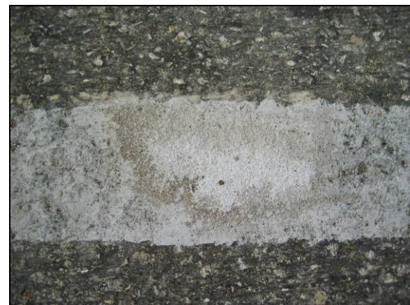
d) Second Installation – Close-Up.
