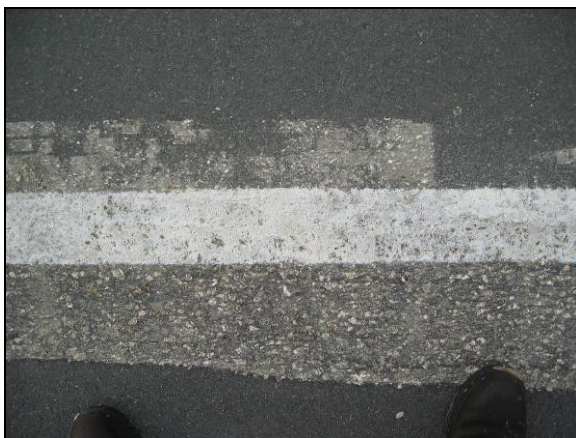
c) Second Installation.
