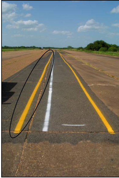
a) Yellow Markings Prior to Removal.
