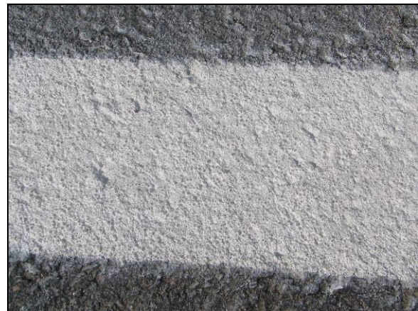
b) First Installation – Close-Up.
