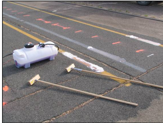
a) Motorized Spray Rig and Brooms.
