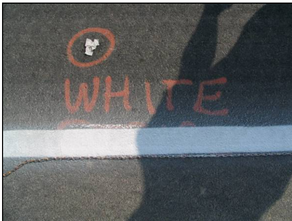
a) First Installation.
