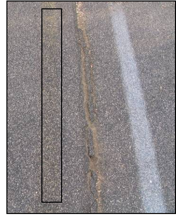
c) Yellow Markings After Removal – Close-Up.
