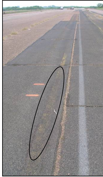
b) Yellow Markings After Removal.
