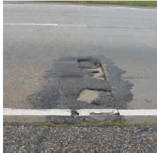
Figure 2-1. Punchouts from TxDOT Distress Manual (TxDOT 2002).
