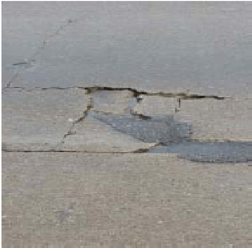
Figure 2-1. Punchouts from TxDOT Distress Manual (TxDOT 2002).
