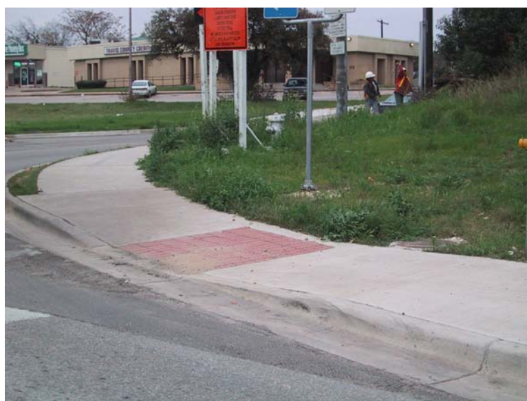
Figure 0-5. Photo of Parallel Curb Ramp.
