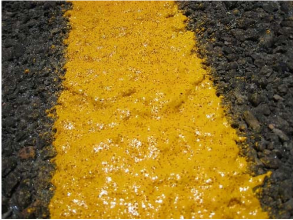
7/31/2007 Initial Install SH 21
