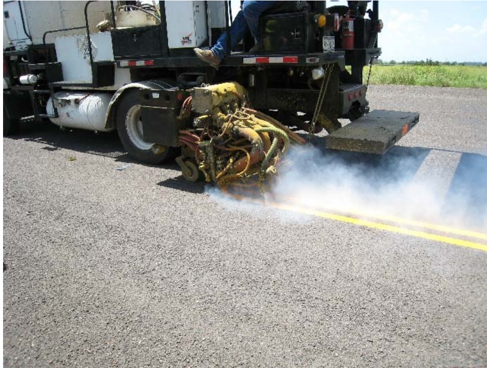
Figure 3-1. SH 21 Lead-Free Thermoplastic Installation.
