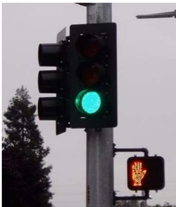
Figure 3-4. Illustrating the Onset of SDW before the Onset of Yellow.
