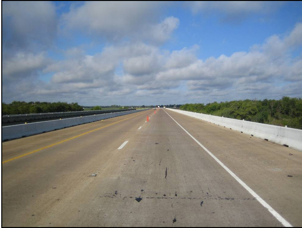
Figure 4-10. Site 5 – SH 21, Bridge over Little Brazos River.
