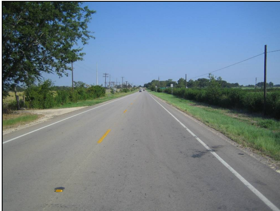
Figure 4-2. Site 1 – FM 46, North of Franklin.
