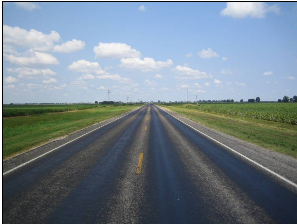
Figure 4-6. Site 3 – FM 50, North of FM 50/FM 60 Intersection.
