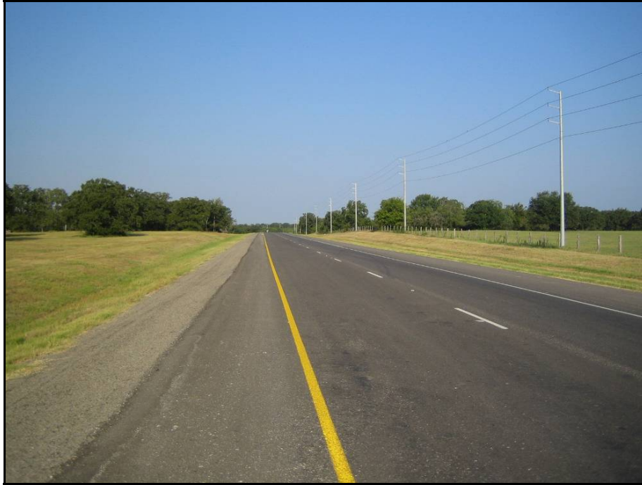
Figure 4-12. Site 6 – SH 40, between SH 6 and Wellborn Road.
