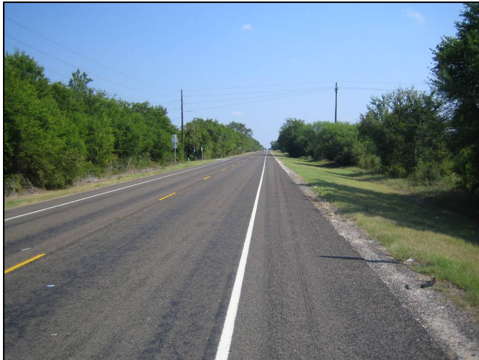
Figure 4-4. Site 2 – FM 39, North of US 190/SH 21 Intersection.
