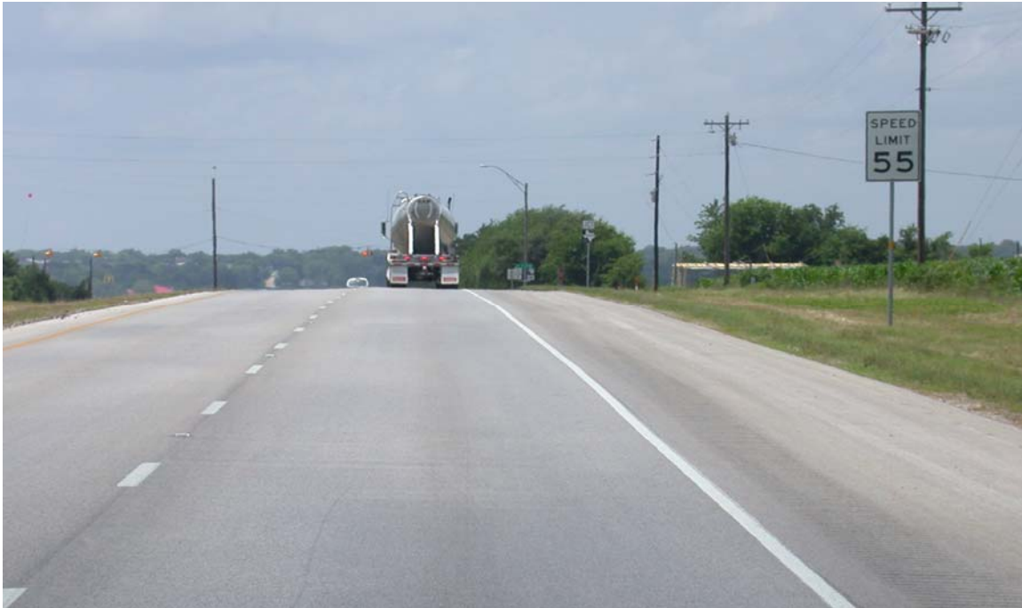
Figure 3-10. Site 5—SH 21, Caldwell Site before 3-Inch Red Border Treatment.
