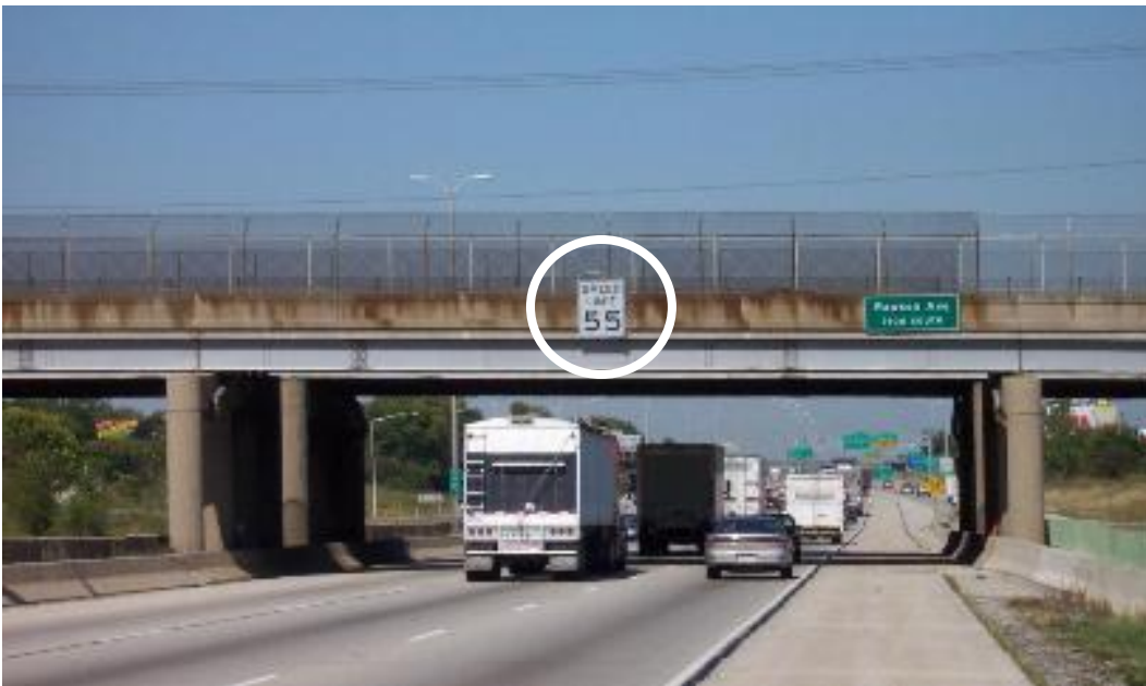
Figure 3-2. Overhead Speed Limit Sign.
