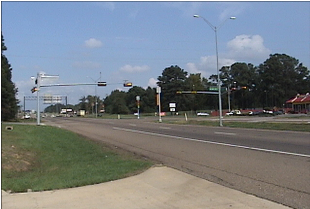
Figure 2-3. US 59 at Emma Lena Way Looking North.
