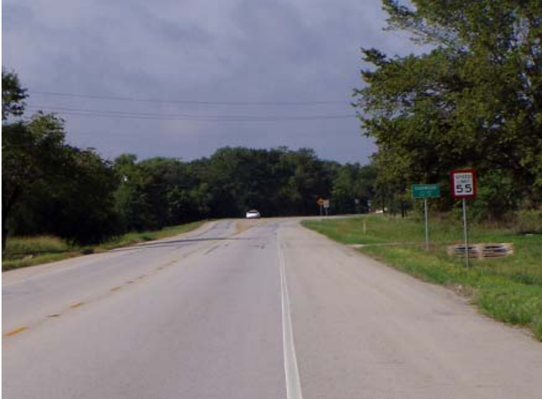
Figure 3-6. Site 3—US 79, Oakwood Site after Modified Red Border Treatment.
