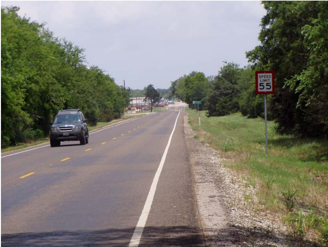
Figure 3-7. Site 4—FM 39, Normangee Site after Modified Red Border Treatment.
