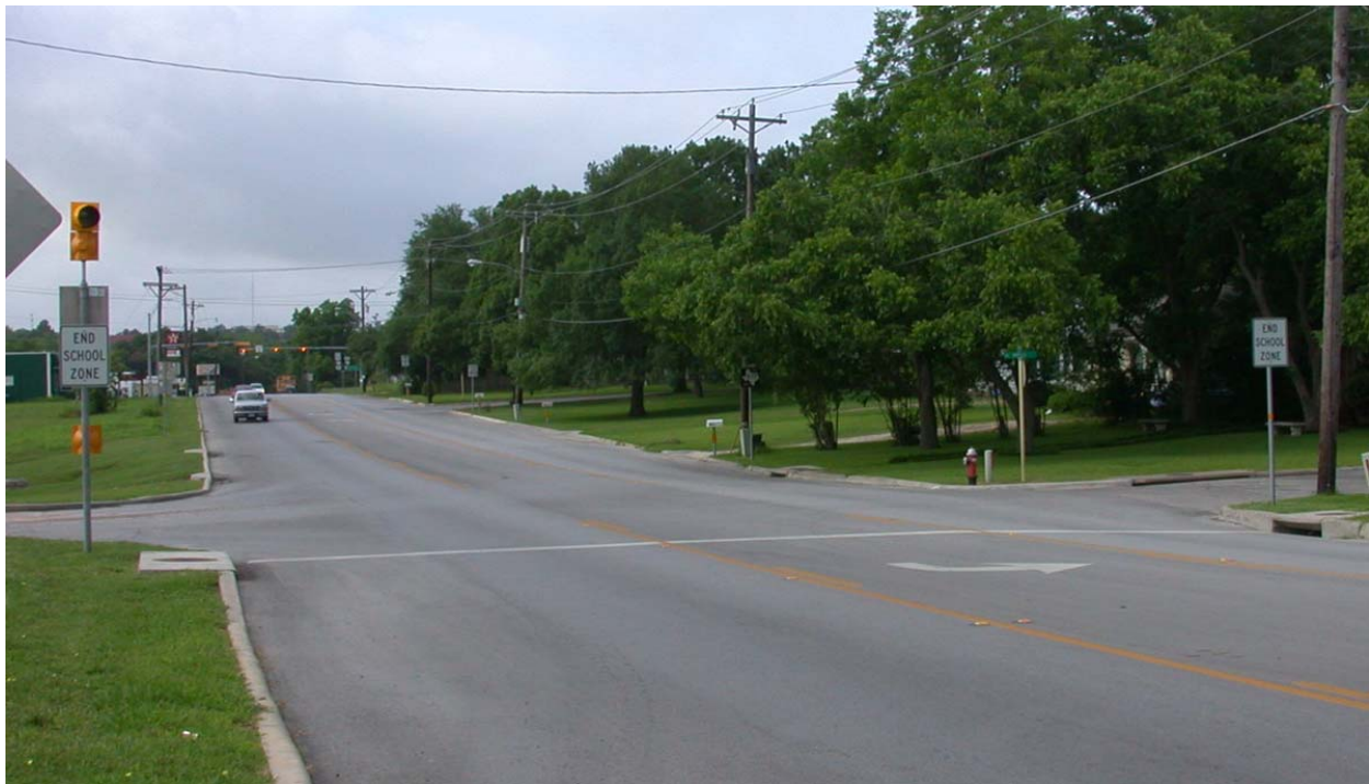
Figure 3-4. Site 2—Brenham High School, School Zone with a Signalized Intersection.
