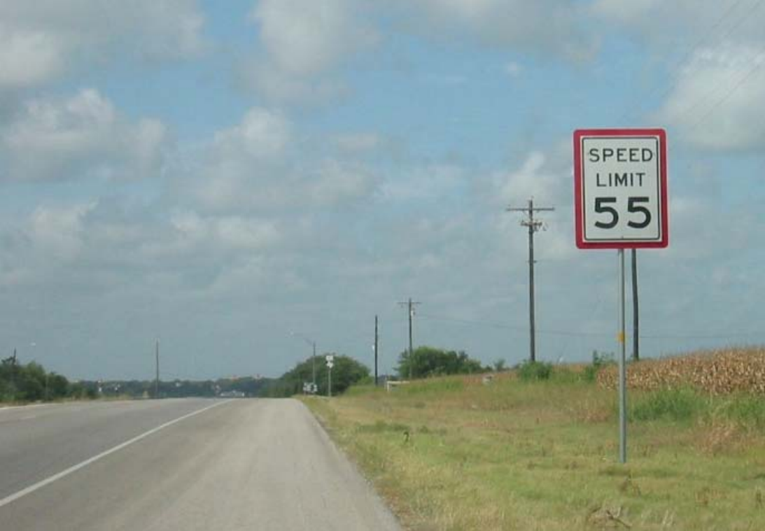
Figure 4-4. Site 1—Caldwell after 3 Inch Red Border Treatment.
