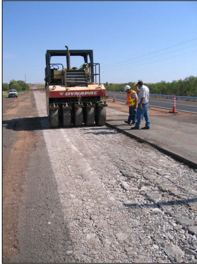
Figure 7.9. Proof Rolling on US 83 from King / Cottle County Line.
