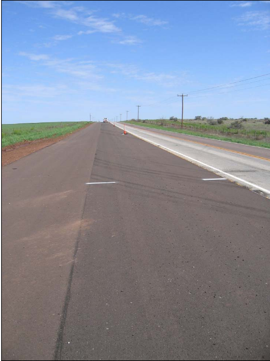
Figure 7.15. Looking North on US 83 SB from STA 1743.
