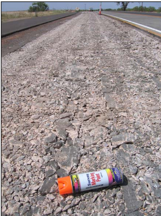
Figure 7.8. Surface and Cross Section Views of Rubblized JCP on US 83.
