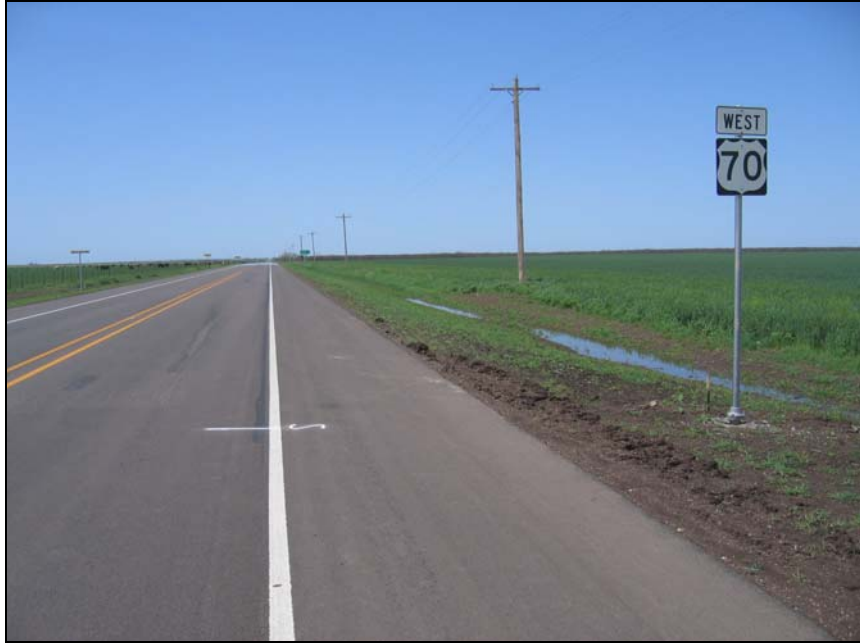
Figure 6.10 Rubblized Section on US 70 WB.
