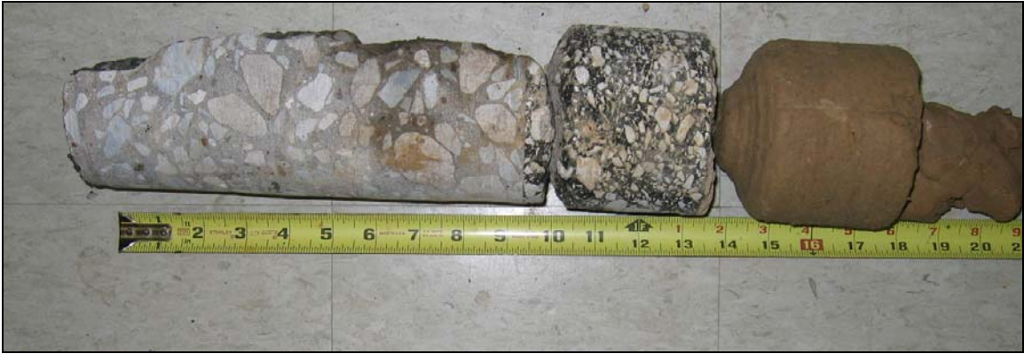
Figure 3.8. Core Collected over Longitudinal Crack. Note the cracking is confined to the concrete layer.
