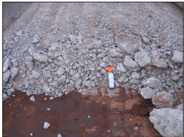
Figure 7.8. Surface and Cross Section Views of Rubblized JCP on US 83.
