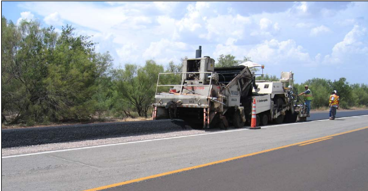
Figure 7.14. Paving Operation on US 83 from King / Cottle County Line.
