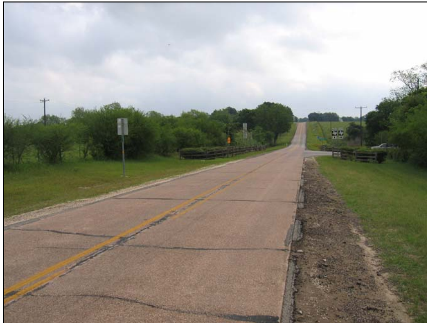
Figure 2.1. JCP Pavement Tested for Suitability for Rubblization.
