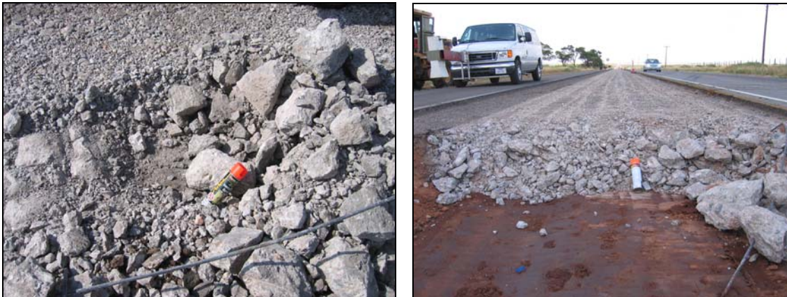
Figure 9.1. Cross Section of Rubblized Layer from MHB (left) and RMI (right).
