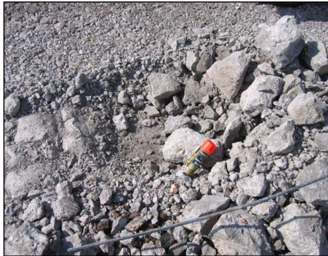
Figure 6.6. Surface and Cross Section Views of Rubblized JCP on US 83.
