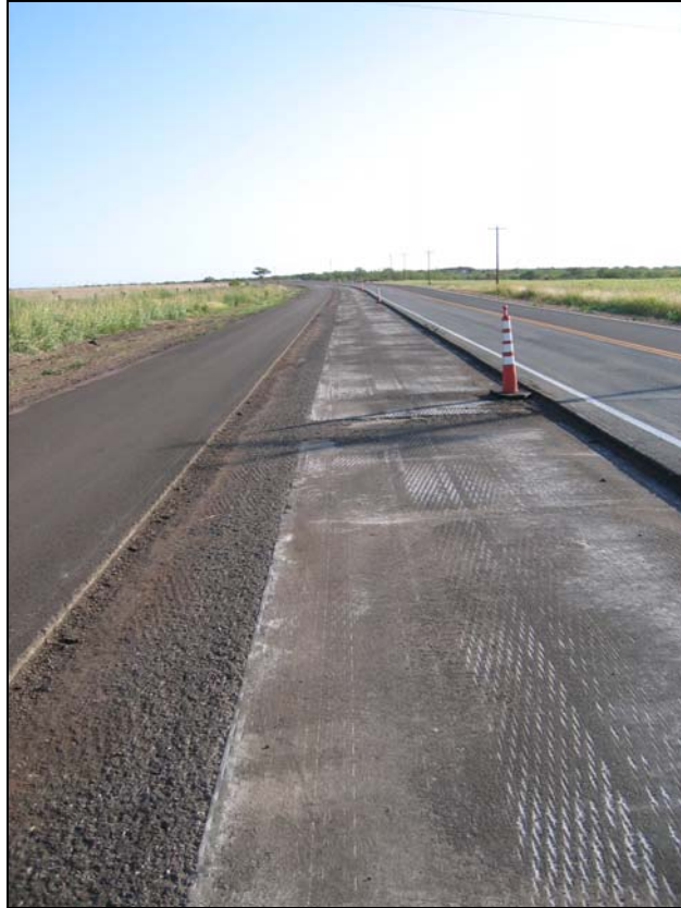
Figure 7.6. Existing Concrete Slabs on US 83 from King/Cottle County Line.
