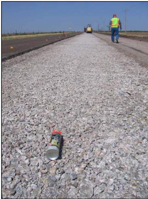
Figure 6.6. Surface and Cross Section Views of Rubblized JCP on US 83.
