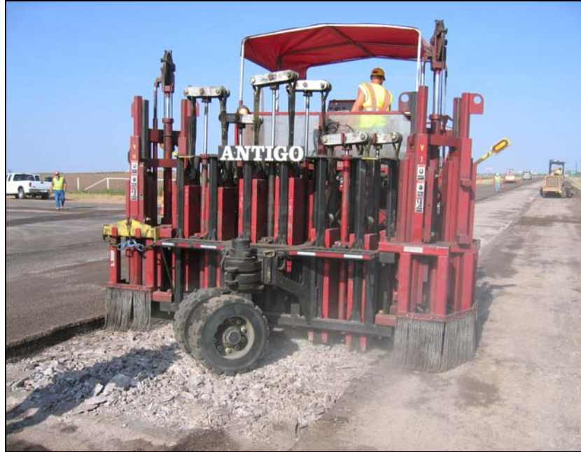
Figure 6.5. Multiple Head Breaker on US 70 in Foard County.
