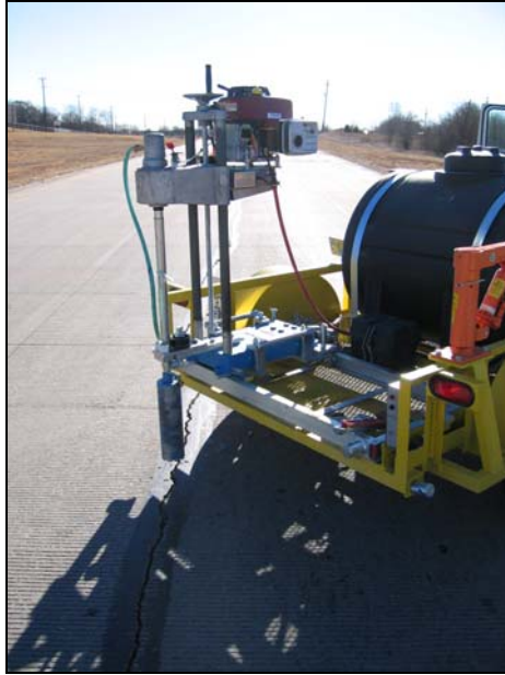
Figure 3.5. Preparing to Core over Longitudinal Crack on Loop 288.
