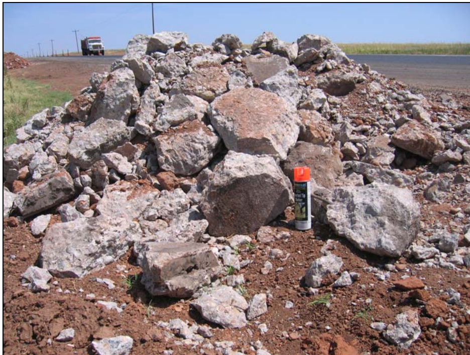
Figure 7.10. Large Particle Sizes Excavated from Removal Location.
