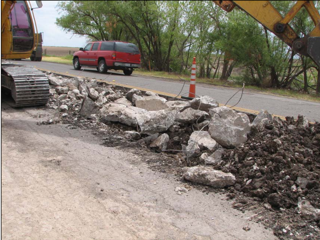
Figure 6.9. Out of Spec Particle Sizes at Failure Location.
