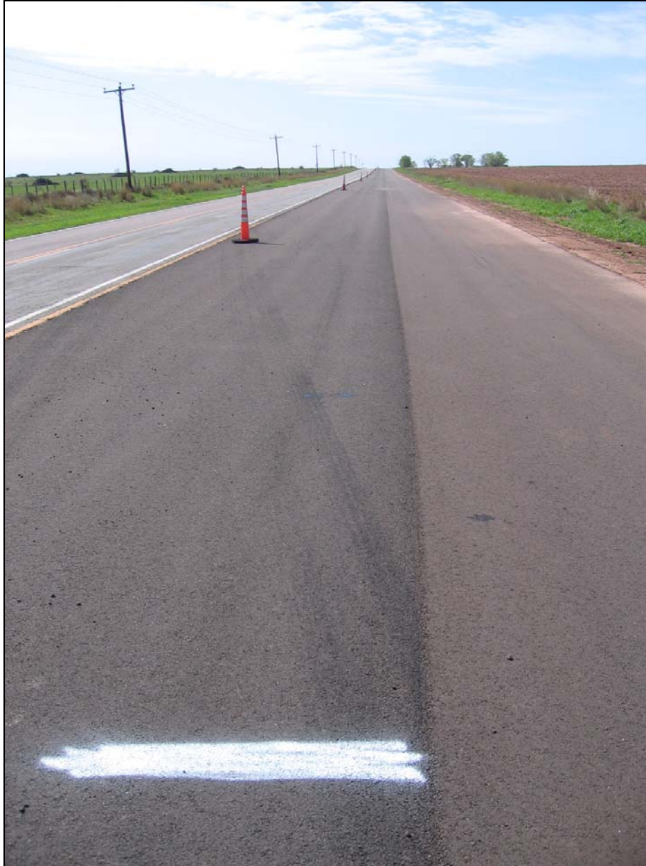
Figure 7.16. Looking South on US 83 SB from STA 1653.
