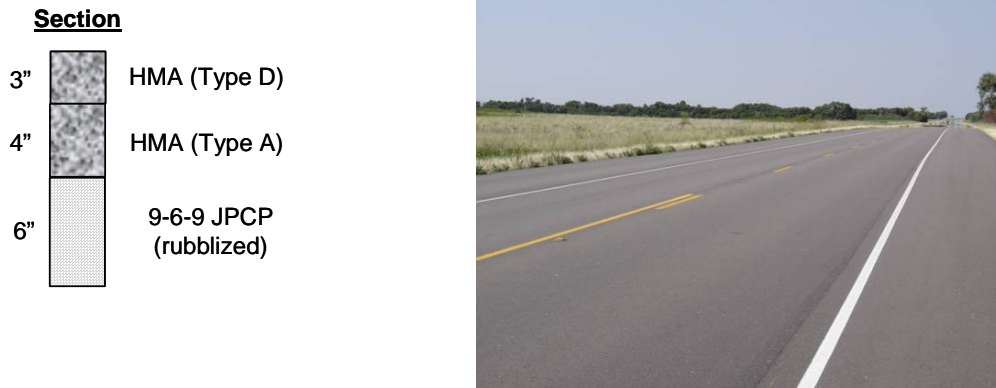
Figure 1.7. US 83 Rubblized Section Constructed in 2003.
