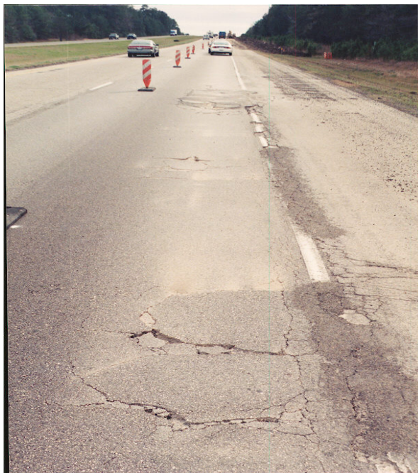
Figure 1.6. Three-Year-Old Crack and Seat Experimental Section on US 59.
