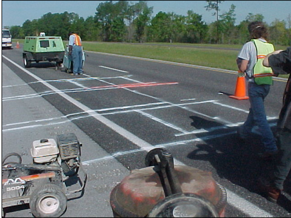
Figure 2. Kistler Sensor Layout before Installation.
