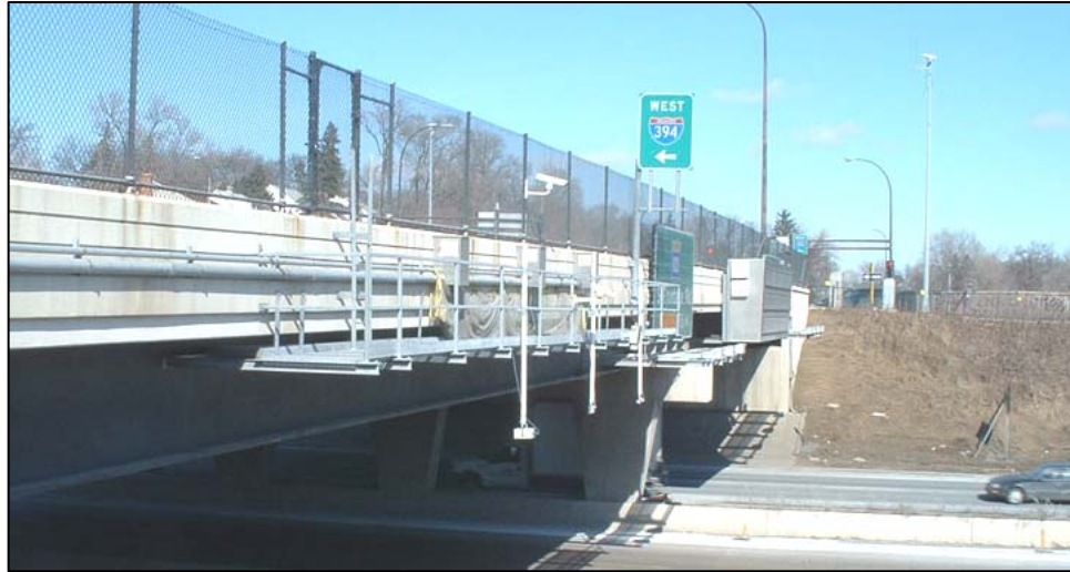
Figure 6. Catwalk for Mounting Detectors Overhead.
