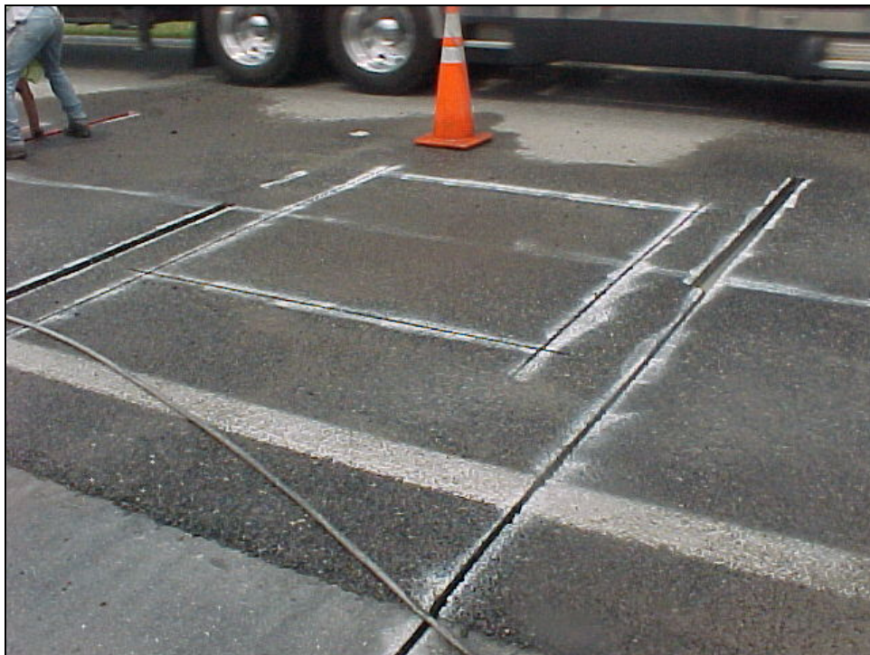
Figure 3. Kistler Sensor Saw Cuts during Installation.
