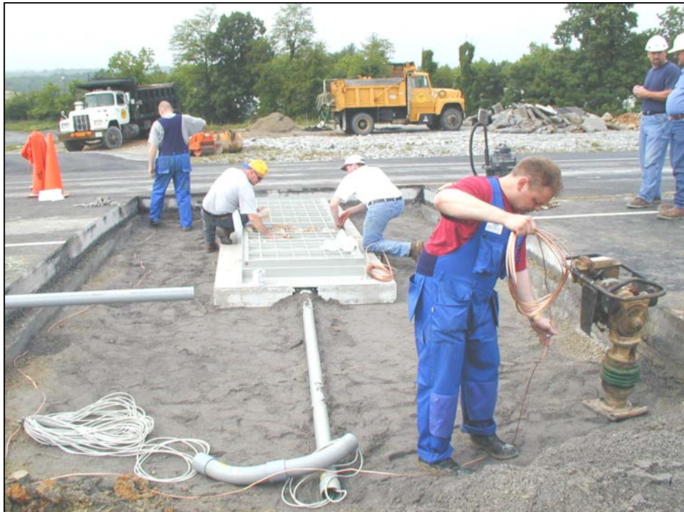
Figure 15. Installation of Omni WIM System at Virginia Tech’s Smart Road.
