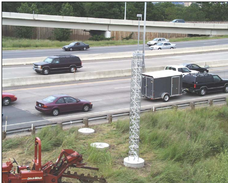
Figure 7. Aluminum Tower for Sidefire Mounting.
