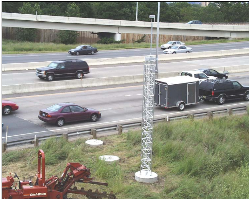
Figure 7. Aluminum Tower for Sidefire Mounting.
