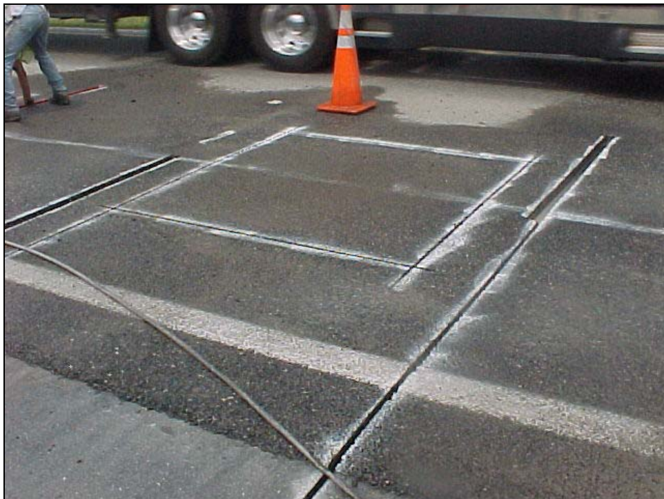
Figure 3. Kistler Sensor Saw Cuts During Installation.
