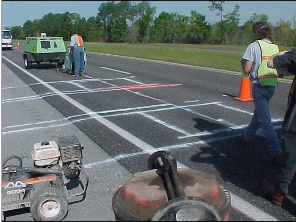
Figure 2. Kistler Sensor Layout Before Installation.
