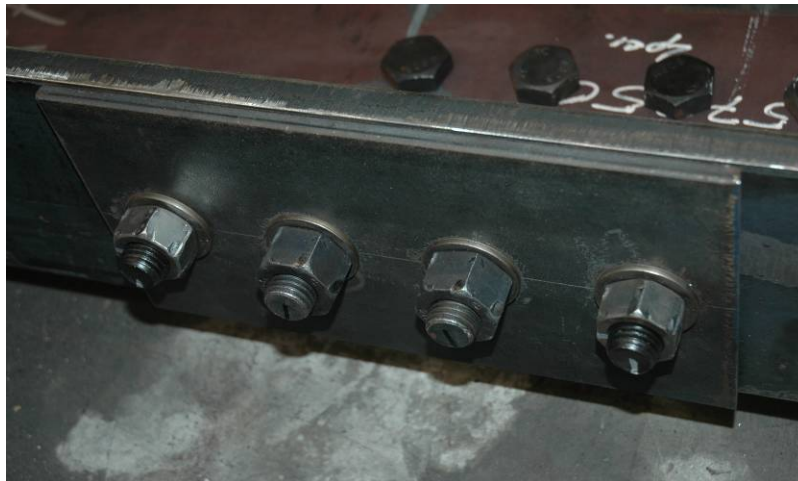
Figure 5-1. Specimen with Bolted Gusset Plate.
