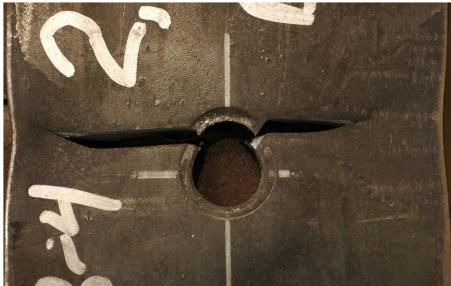
Figure 5-8. Typical Crack Orientation for Thin Plates (<1.0 Inches) with a Gusset Plate (Specimen B-4).
