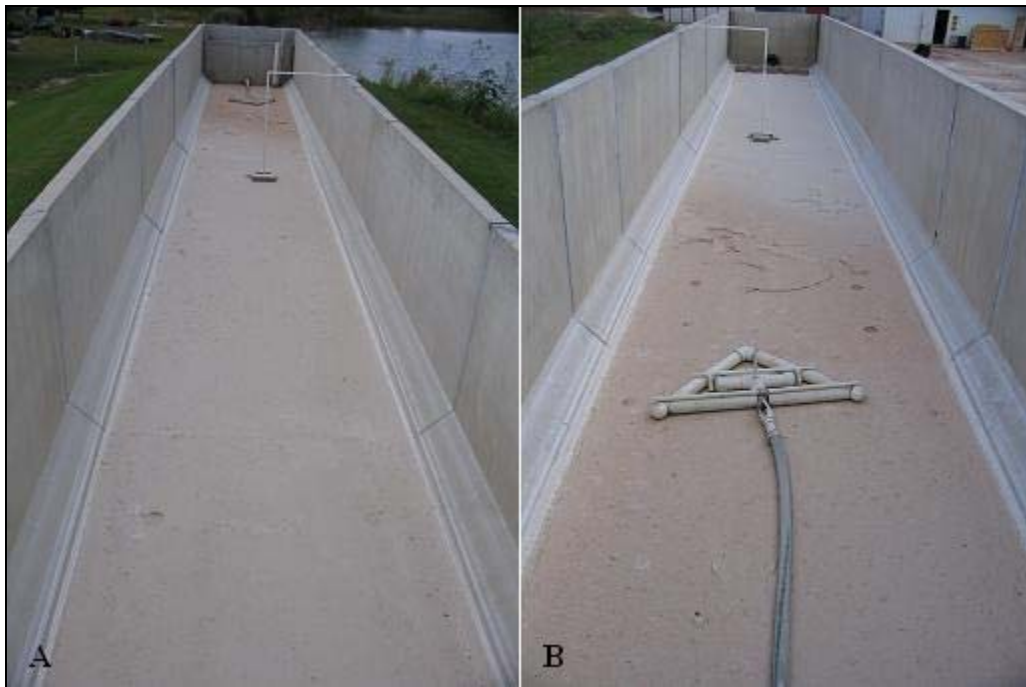
Figure 2.3. View of Sedimentation Tank Before Outlet Relocation.
