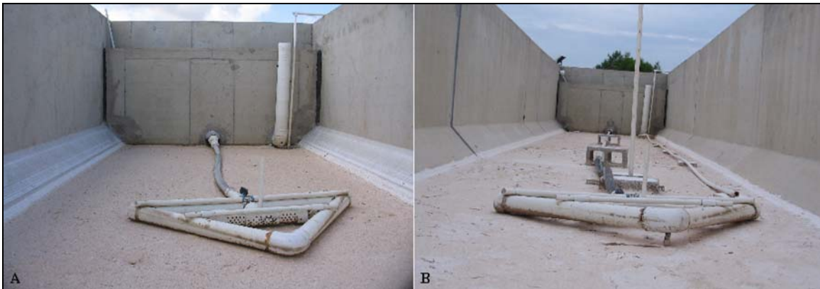
Figure 2.4. View of Fixed and Floating Outlet. A. Outlets at End. B. Outlets in Middle.
