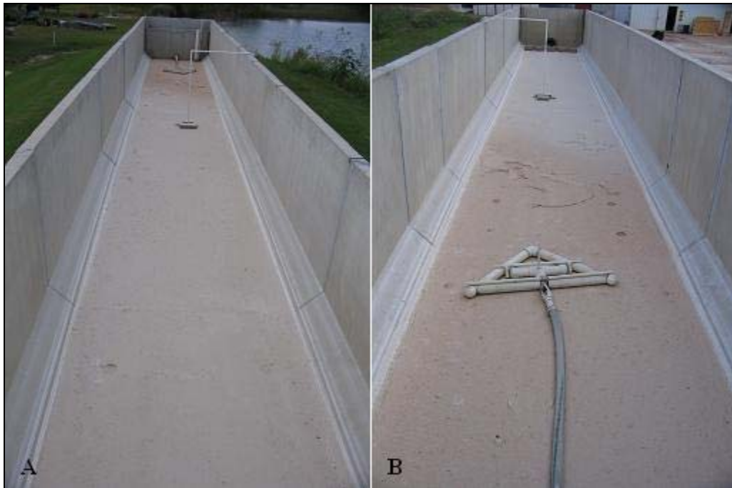
Figure 4.3. A. View from Upstream. B. View from Downstream.
