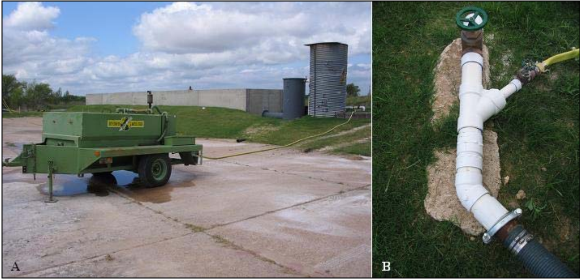
Figure 4.1. A. Hydroseeder for Making Slurry. B. Point of Injection into Main Line.
