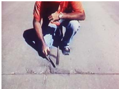
Detecting delaminated areas in concrete bridge decks
