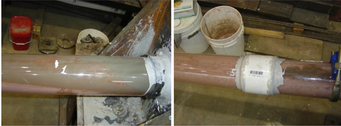
Figure B-10. Repair Grouted Ducts of Specimen VG-C3-1.
