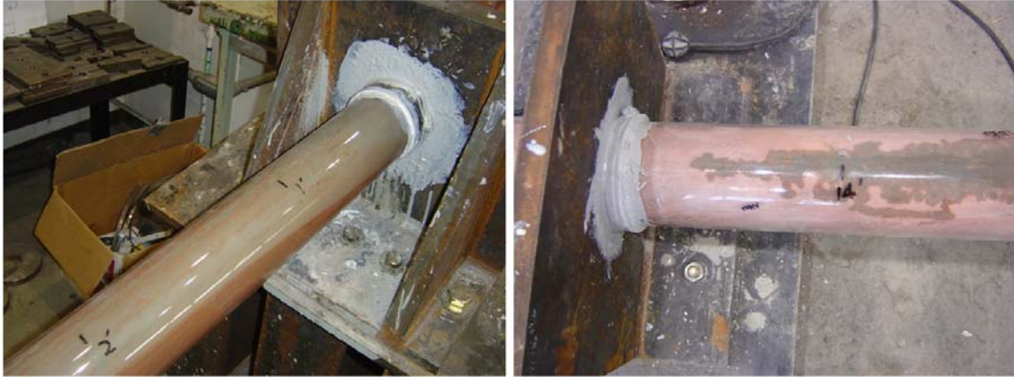
Figure B-34. Repair Grouted Ducts of Specimen PVG-C1-2.
