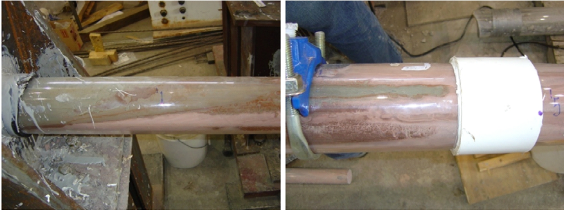
Figure B-19. Repair Grouted Ducts of Specimen PG-C2-1.
