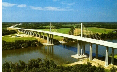
Figure 2-7. Varina-Enon Bridge, over the James River, Virginia (Roadstothe future 2009).
