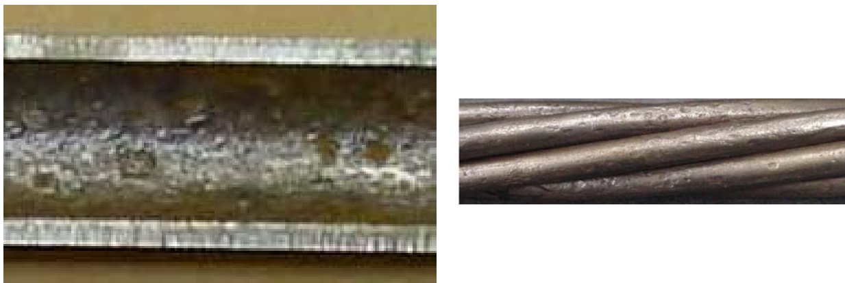
Figure 2-9. Pitting Corrosion on ASTM A 53 Pipe and ASTM A 416/A 416M-99 Strand Due to Coupled Galvanic- and Chloride-Induced Corrosion ( FDOT 2002 ).
