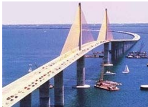
Figure 2-5. Bob Graham Sunshine Skyway Bridge, Tampa Bay, Florida ( Wikipedia 2009 ).
