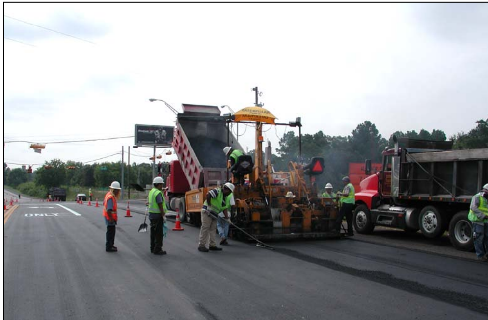
Figure 1.15. Placement Operation of Superpave D on Business 290.
