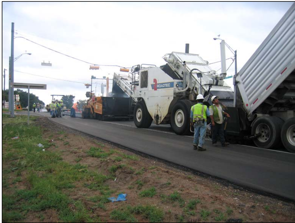
Figure 1.17. Placement Operation of Type D Mix on Business 290.
