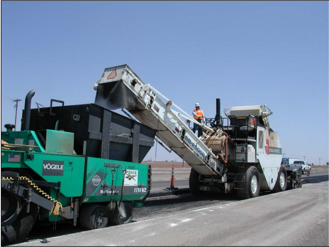
Figure 1.9. Placement Operation on IH 20 1 inch Superpave.
