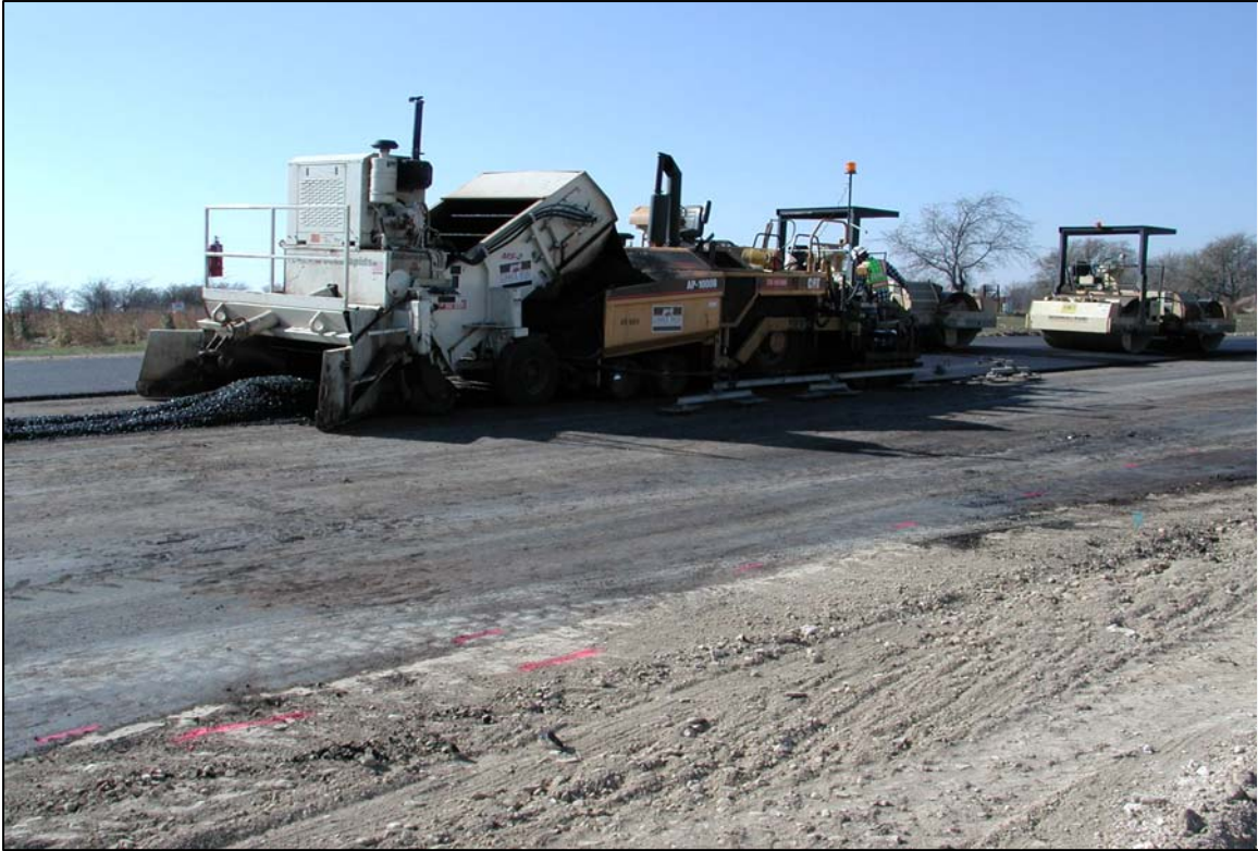
Figure 1.5. SH 114 ¾ inch SFA Placement Operation, Day 1.
