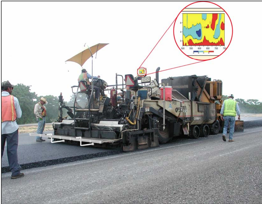
Figure 3.1. Concept Infrared Sensor Bar Mounted to Paver for Implementation.
