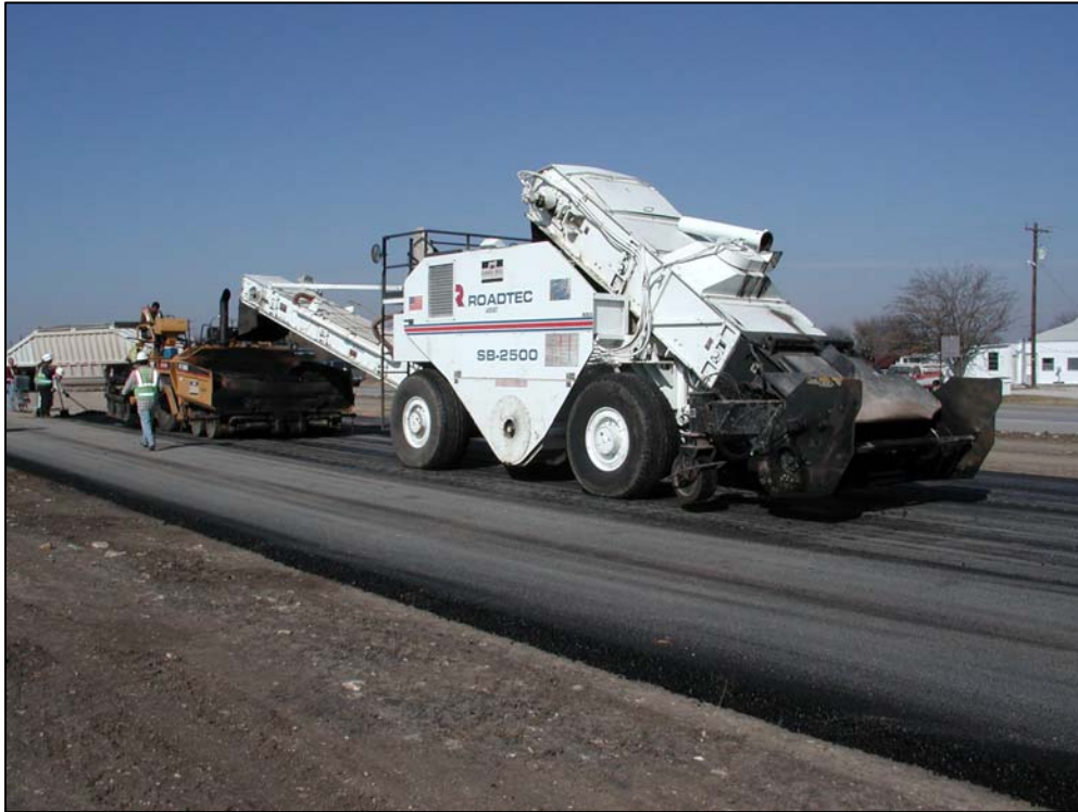
Figure 1.7. SH 114 ¾ inch SFA Placement Operation, Day 2.
