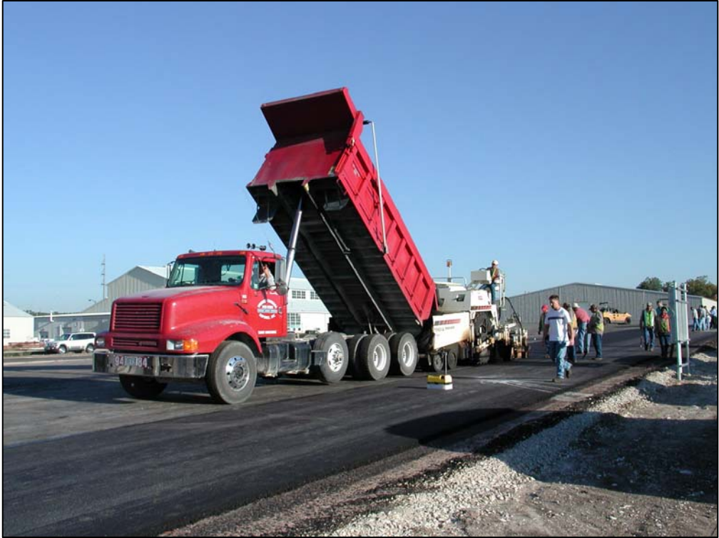
Figure 1.3. Placement Operation at MLS Test Site.
