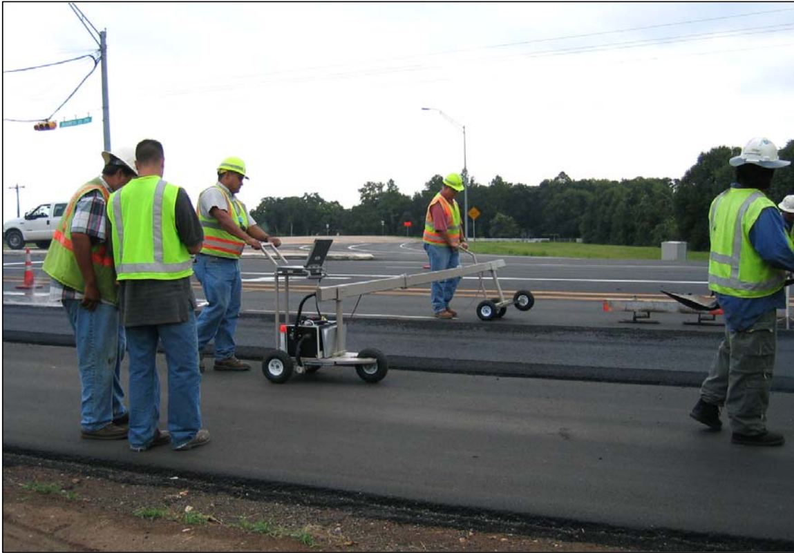
Figure 1.12. Second Generation Infrared Sensor Bar on Paving Project.
