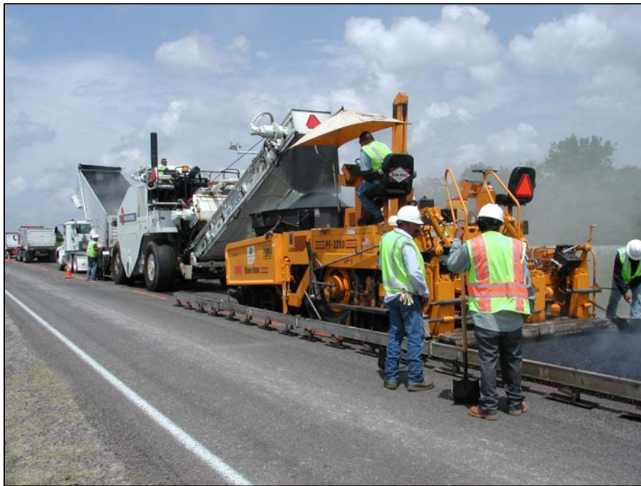
Figure 1.13. Placement Operation on US 90 in Brookshire, Texas.
