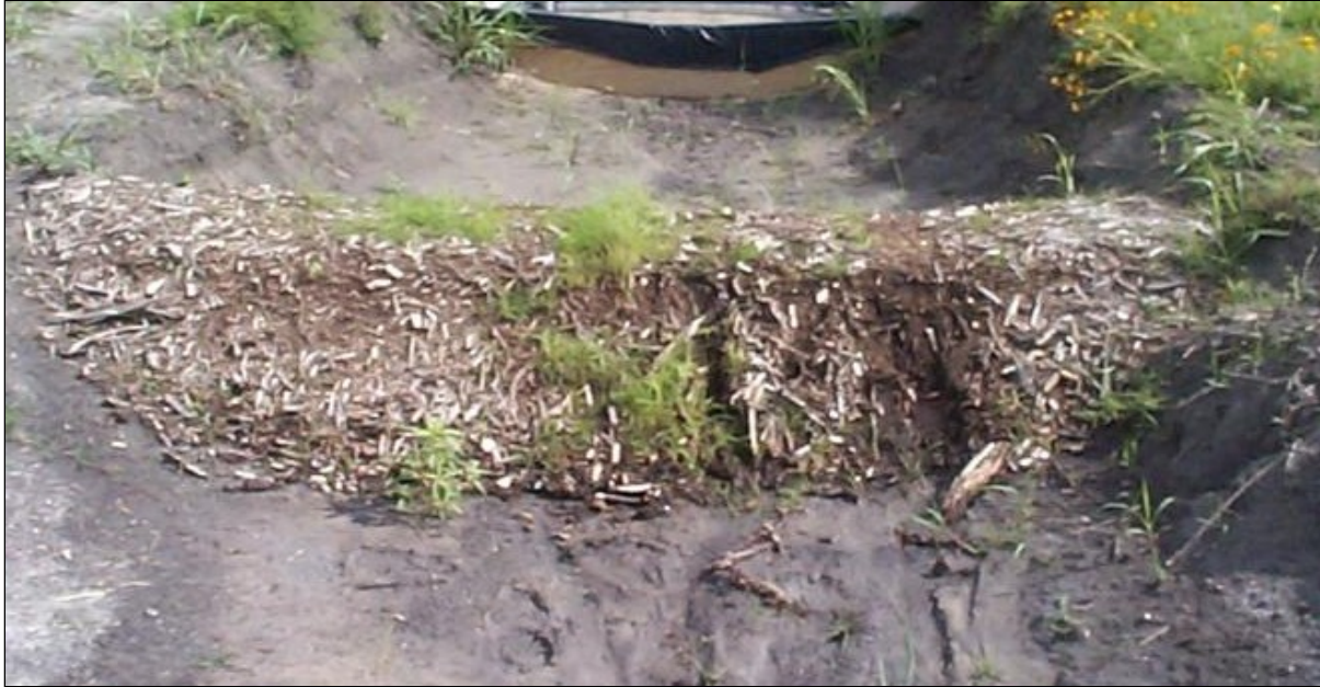
Figure 4.11. Composted Biosolids Berm Showing Minor Damages to the Leading Face.
