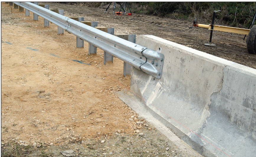
TL-2 Transition prior to Testing.
