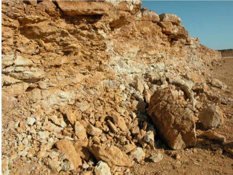
Figure 2. Ten-Foot Working Face at the Baird Quarry Illustrating Resistant Limestone Intercalated with Fissile Shale and Sandstone Lenses.
