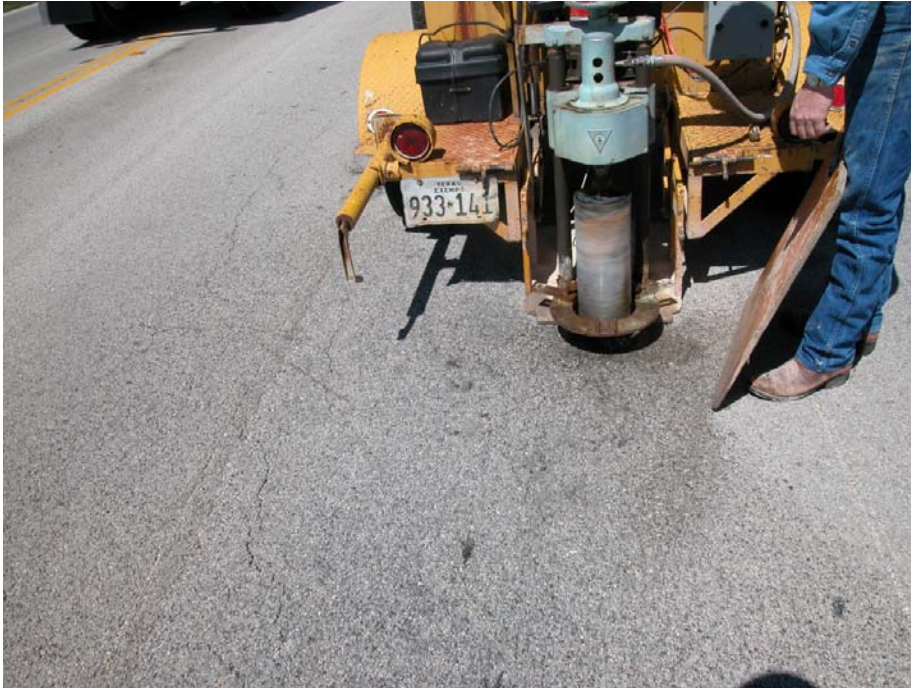
Figure 3. Drilling Cores from US-84.
