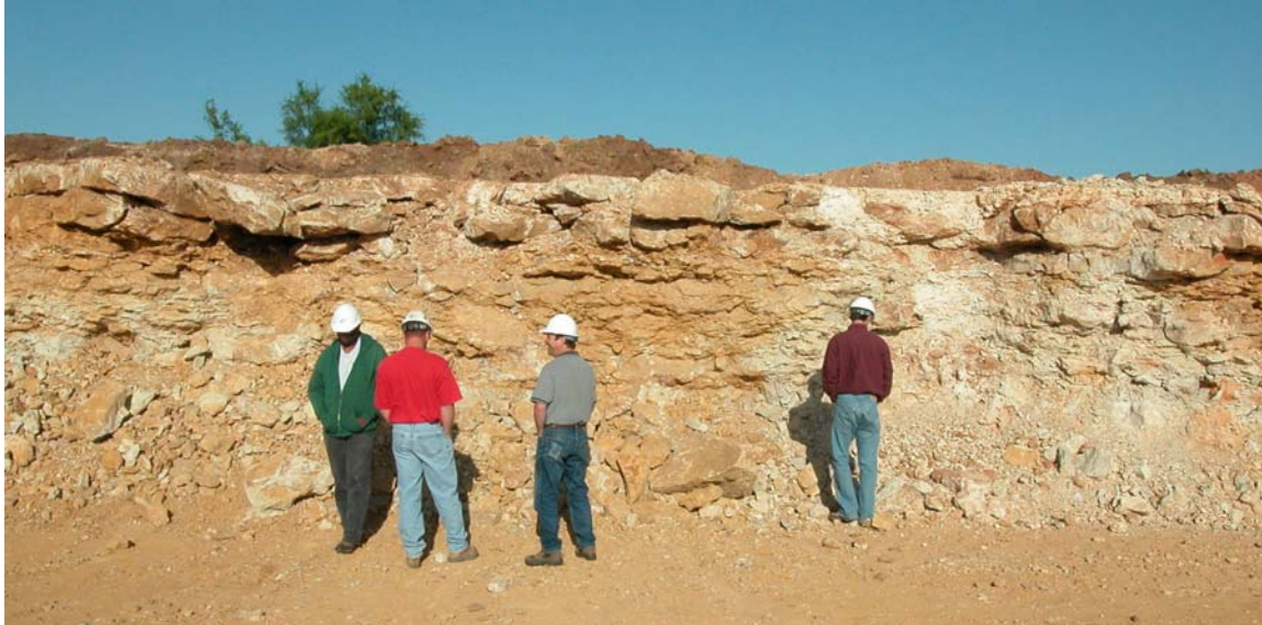
Figure 1. Working Face at the Baird Quarry Shows a Thin (2 foot) Resistant Unit at Top.
