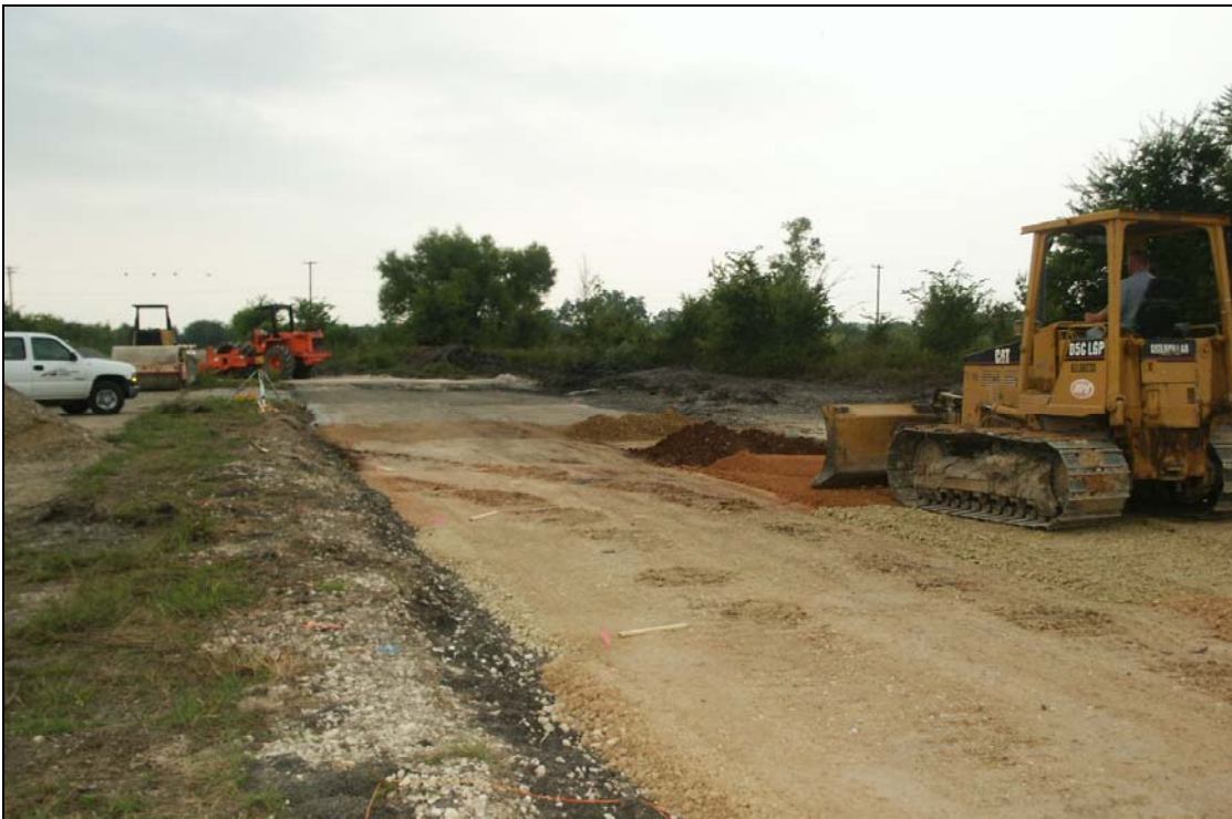
Figure 4.11. Construction of Different Base Sections.
