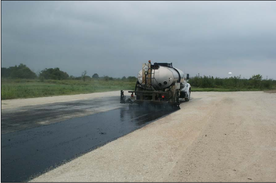
Figure 4.12. Application of Surface Treatment on Sandy Site.
