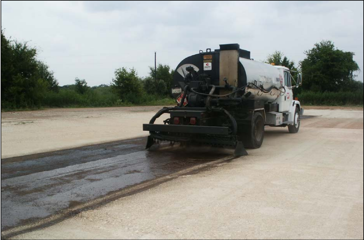
Figure 4.7. Prime Coat Application to the Sandy Site Base Sections.
