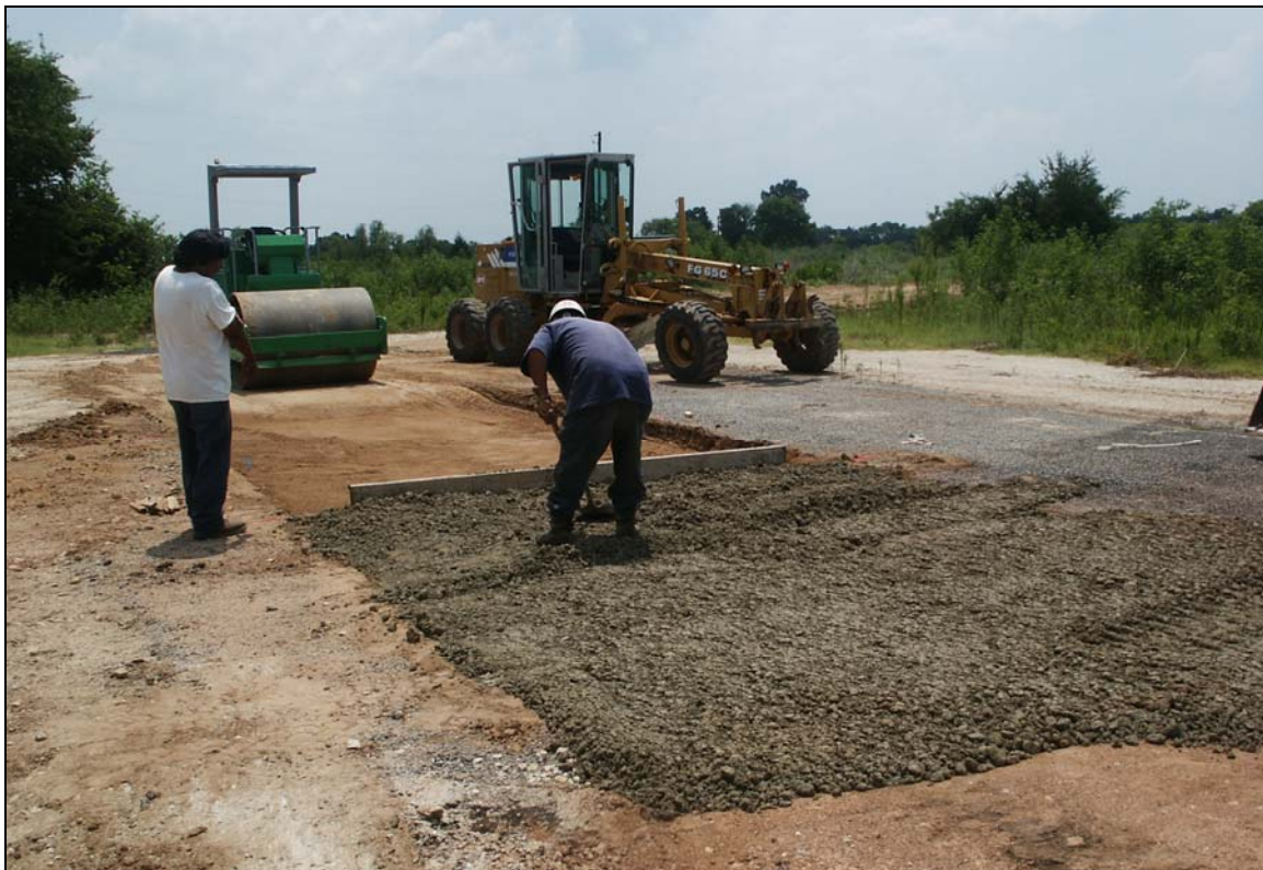
Figure 4.20. Placement of Cement-Treated Grade 2 Base Material.
