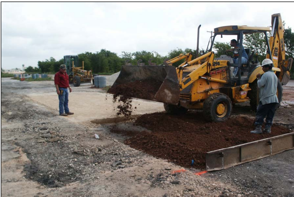
Figure 4.15. Placement of Uncrushed Gravel Treated with 2 Percent Lime.
