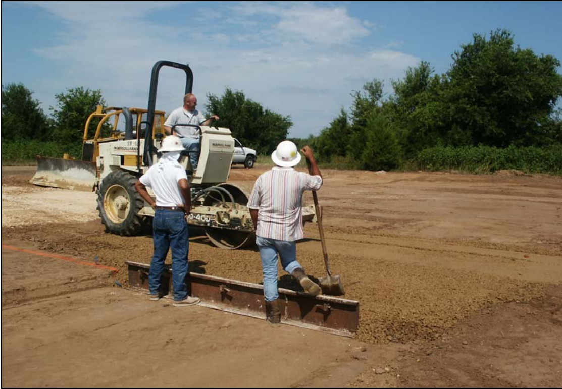
Figure 4.6. Placement of First 6-inch Lift (of 12-inch Thick Section) of Sandstone.
