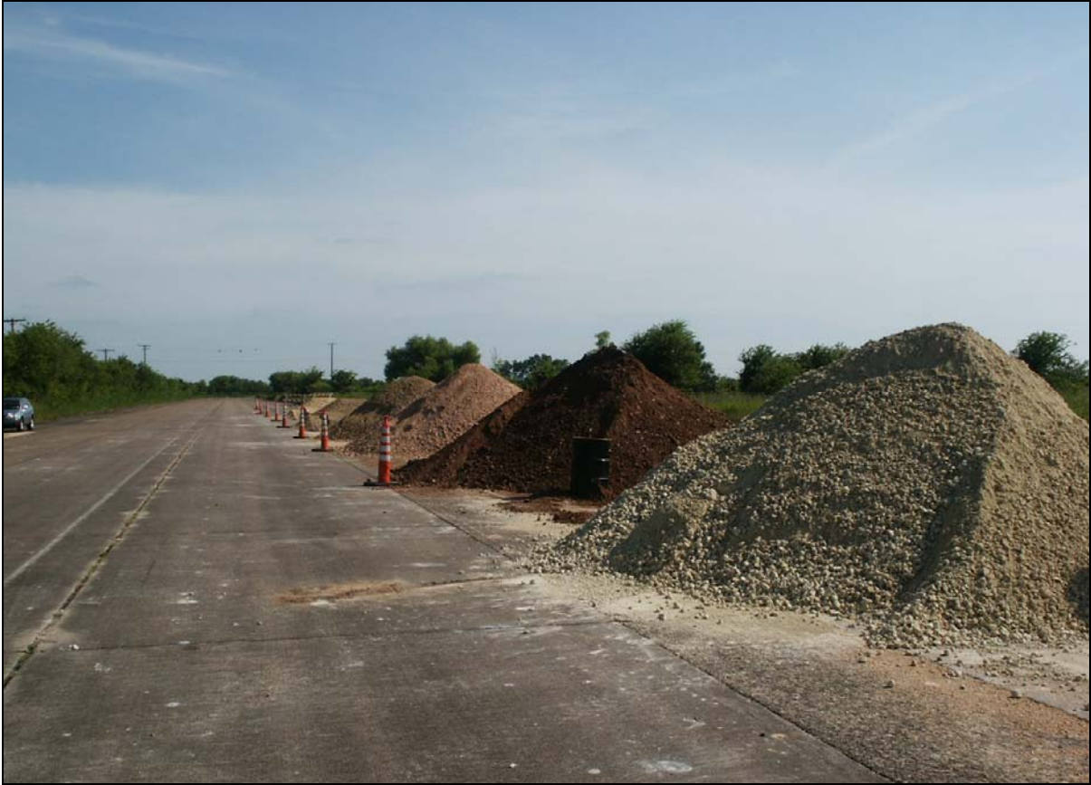
Figure 4.1. Stockpiled Base Materials at Riverside Campus on Taxiway 7.
