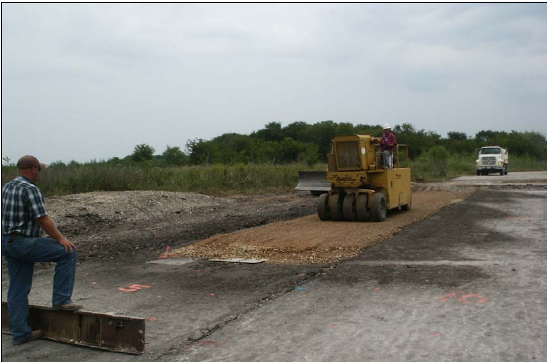
Figure 4.9. Placement of First Base Material on Clay Subgrade.
