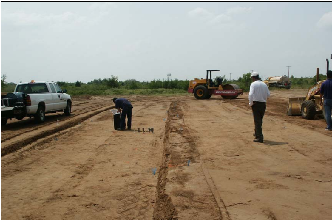
Figure 4.3. Finished Subgrade at Sandy Site.
