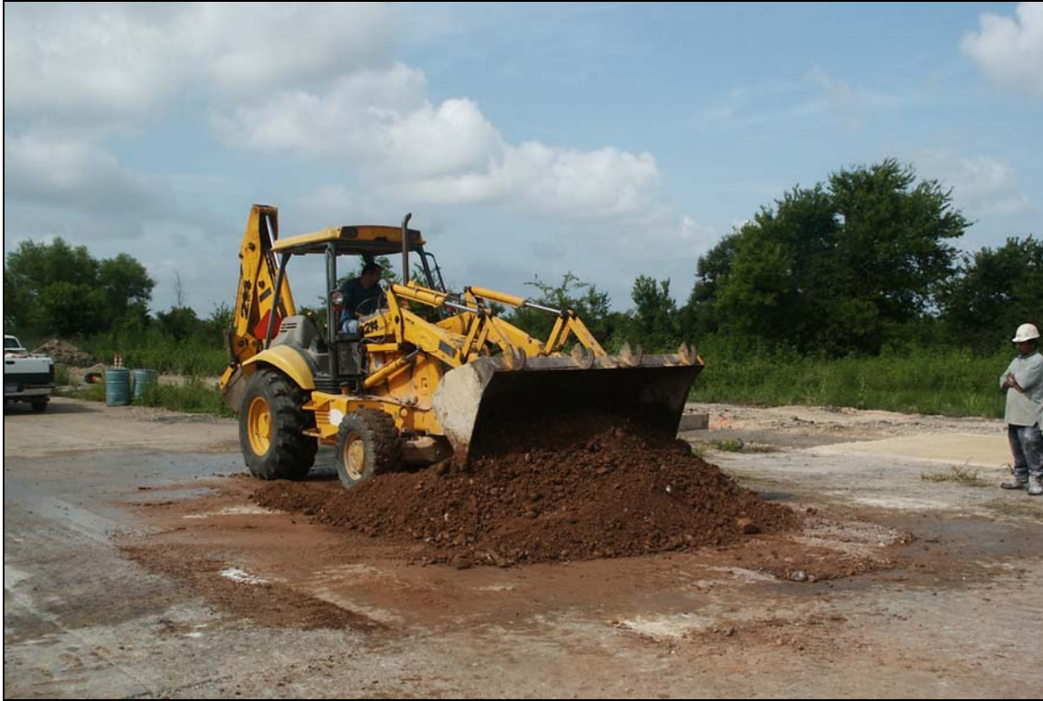
Figure 4.14. Mixing Uncrushed Gravel with Lime on Concrete Pad.
