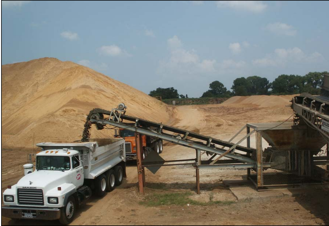
Figure 4.19. Plant Mixed Grade 2 Base to be Hauled to Test Site.
