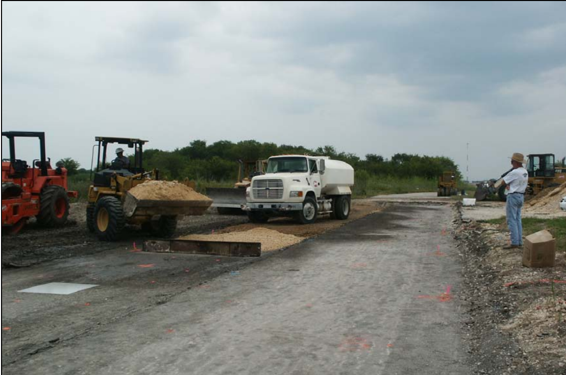
Figure 4.10. Placement of Second Base Material on Clay Subgrade.
