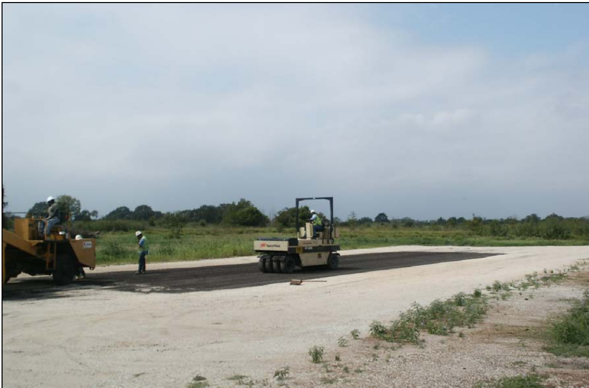
Figure 4.13. Completed Surface Treatment on Sandy Site.
