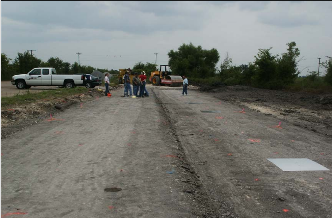
Figure 4.8. Prepared Clay Subgrade.
