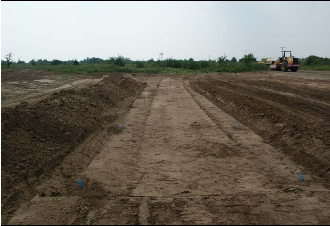
Figure 4.2. Preparation of Sandy Subgrade.
