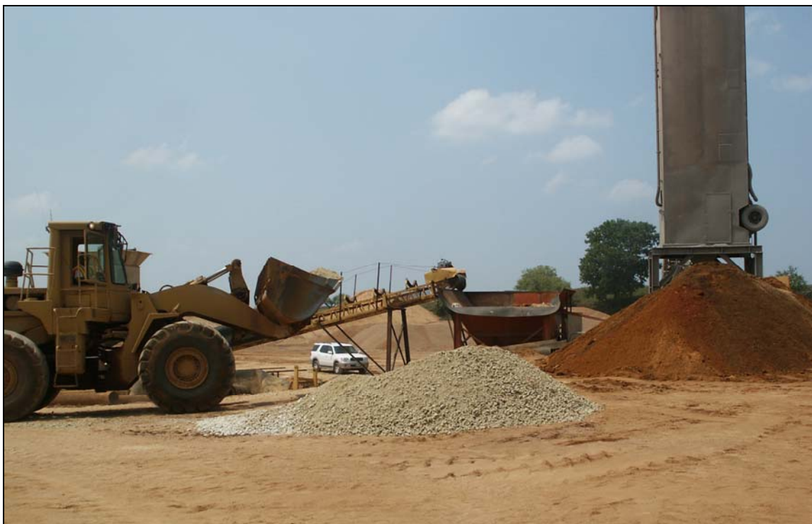
Figure 4.18. Transferring Stockpiled Grade 2 into Pugmill Hopper with Front-End Loader.
