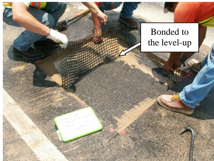
Figure 17. Photograph of a Trench on IH 35E.
