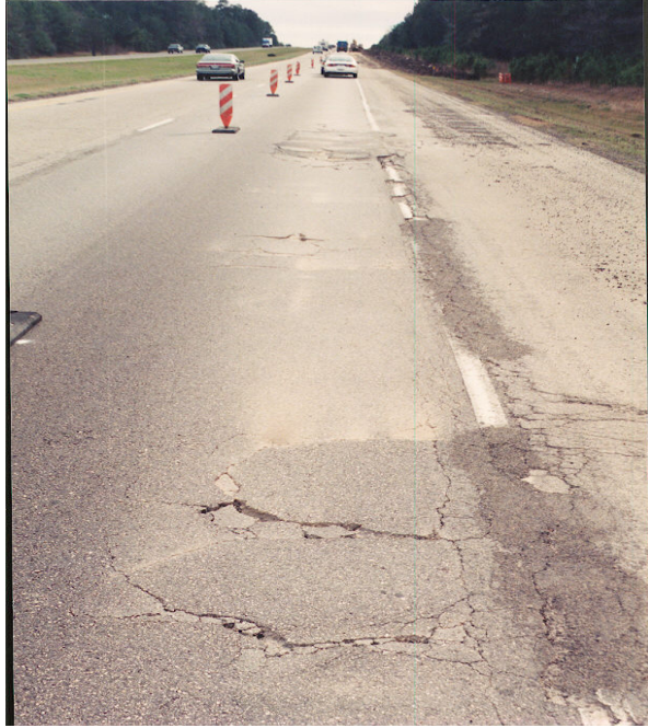
b) Section R2 Crack and Seat (2000)
