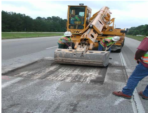
Figure 14. Sampling Materials from Section R3 on US 59.
