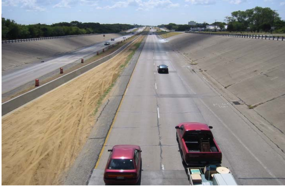
Figure 51. View of the Section of US 175 that Received Both the GlasGrid® and Strata® Treatment in December 2003.
