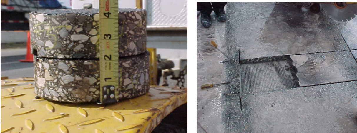
Figure 35. IH 45 Field Cores and Trench from the Failed GlasGrid® Section.
