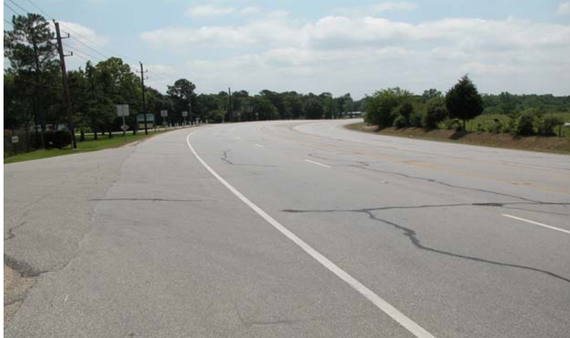
Figure 30. Petromat Section on FM 2920 after Four Years of Service.
