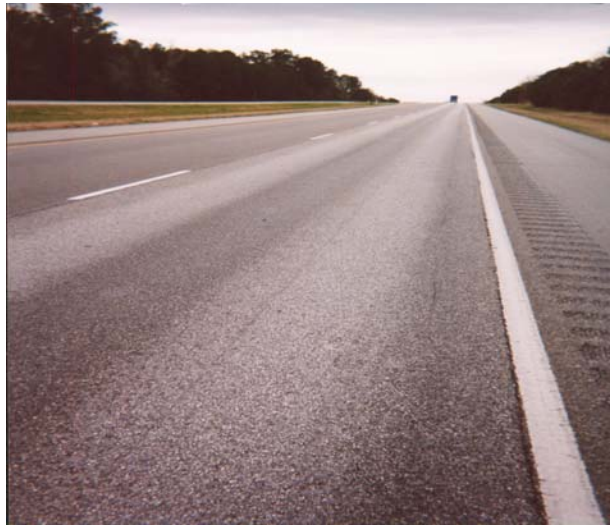
c) Flexible Base Overlay (section R3) (2000)
