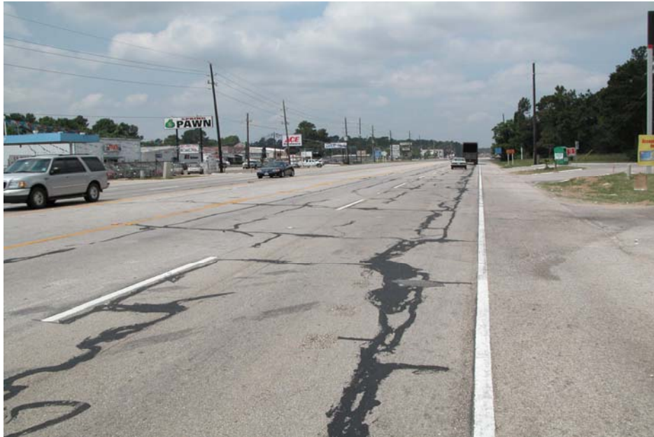
Figure 29. GlasGrid® Section on FM 2920 – Note Deterioration in Wheel Paths.
