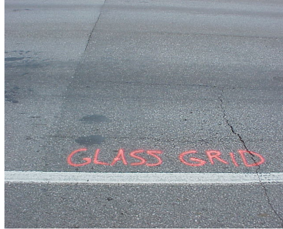
b) Transition from Crumb Rubber to GlasGrid® Section
