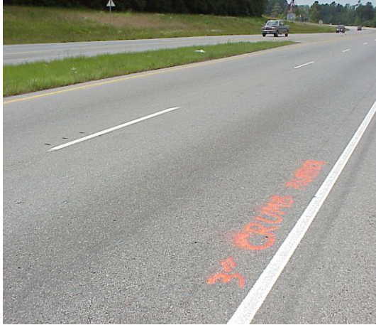
a) Crumb Rubber after 8 Years, Excellent condition
