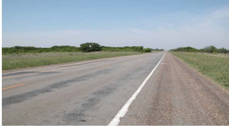
Figure 52. Rubblization Site on US 83 South of Childress.
