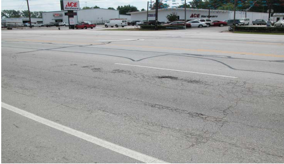
Figure 28. GlasGrid® Section on FM 2920 after Four Years of Service.
