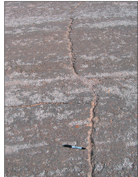
3a. Sample Cracking in Microcracked Pavement (top)
