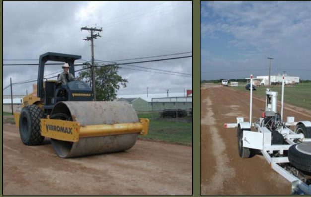
Microcracking in progress with the vibratory roller. TxDOT's FWD can serve as the control mechanism to determine when to stop rolling by measuring the reduction in average base modulus.
