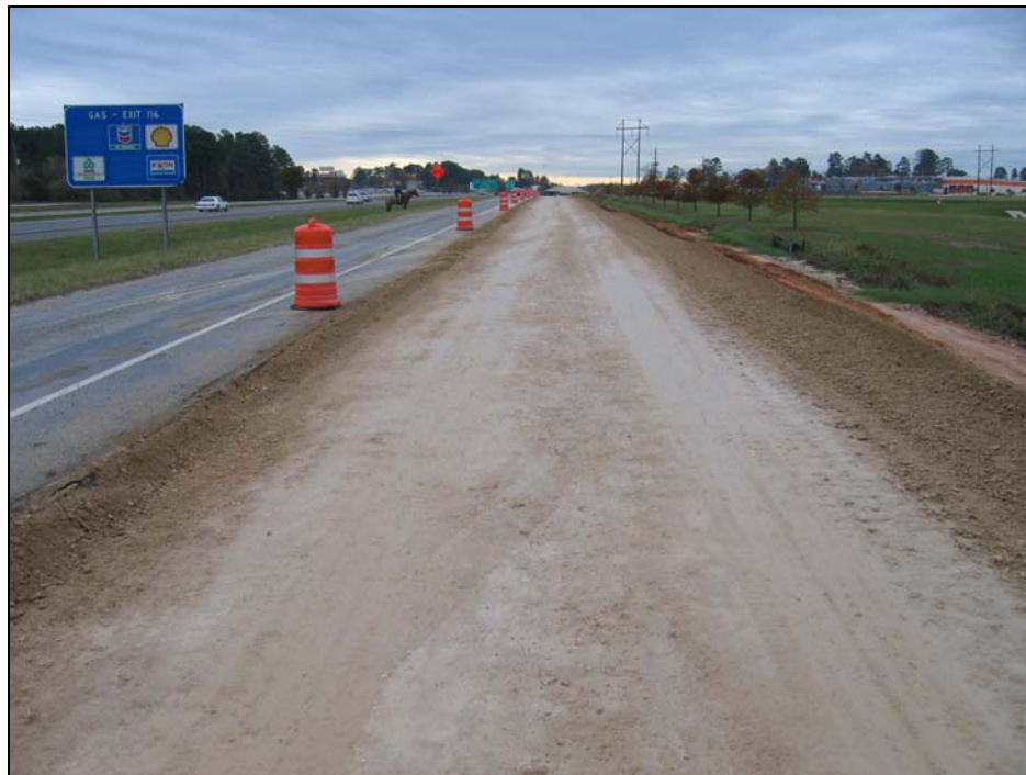
Figure 3.2. Looking South on the SB IH 45 Frontage Road Project.
