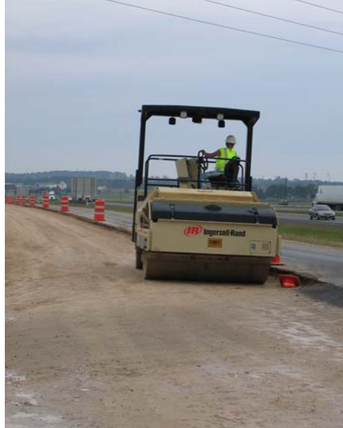
Figure 3.4. Microcracking IH 45 SB OL on December 6, 2004.
