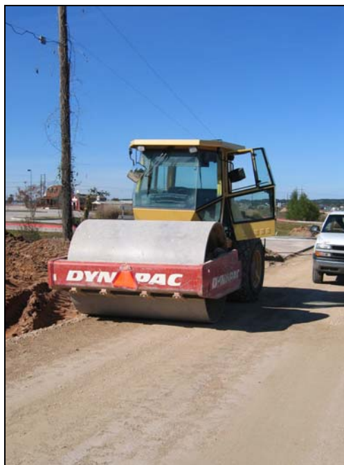
Figure 3.5. Microcracking IH 45 SB OL on December 7, 2005.
