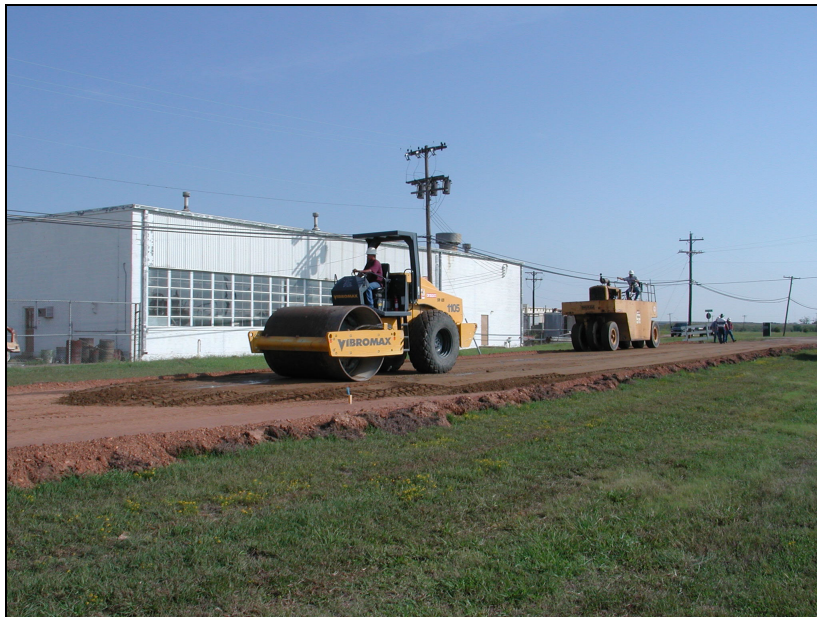
Figure 5.4. Rolling in CTB at Riverside Campus.
