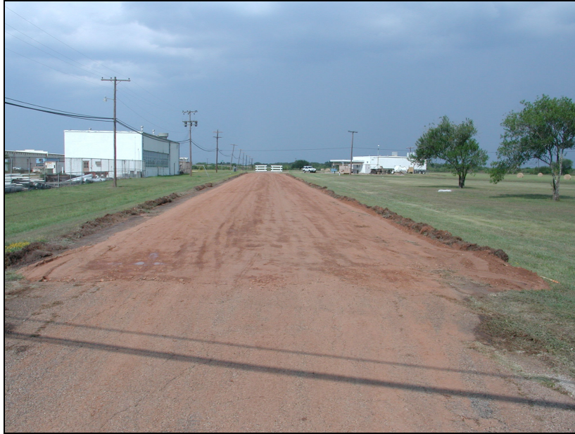
Figure 5.3. Prepared Subbase at Riverside Campus.
