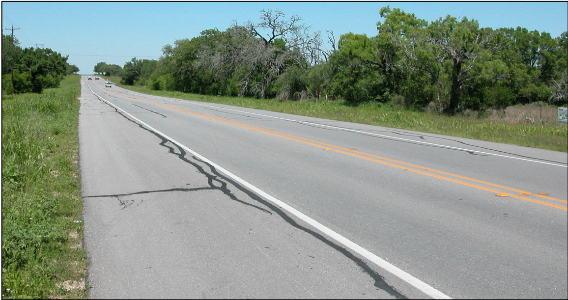
Figure 4.5. SH 16 Test Sites 1 (left lane) and 2 (right lane) on April 13, 2004.
