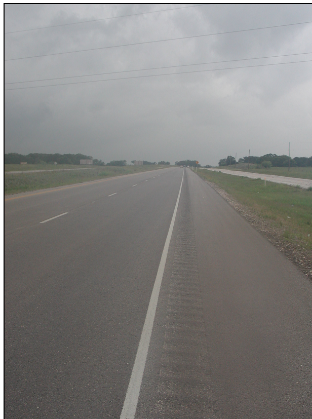
Figure 3.1. NB CTB Site on SH 47 from STA 1362+60 to 1346+76.
