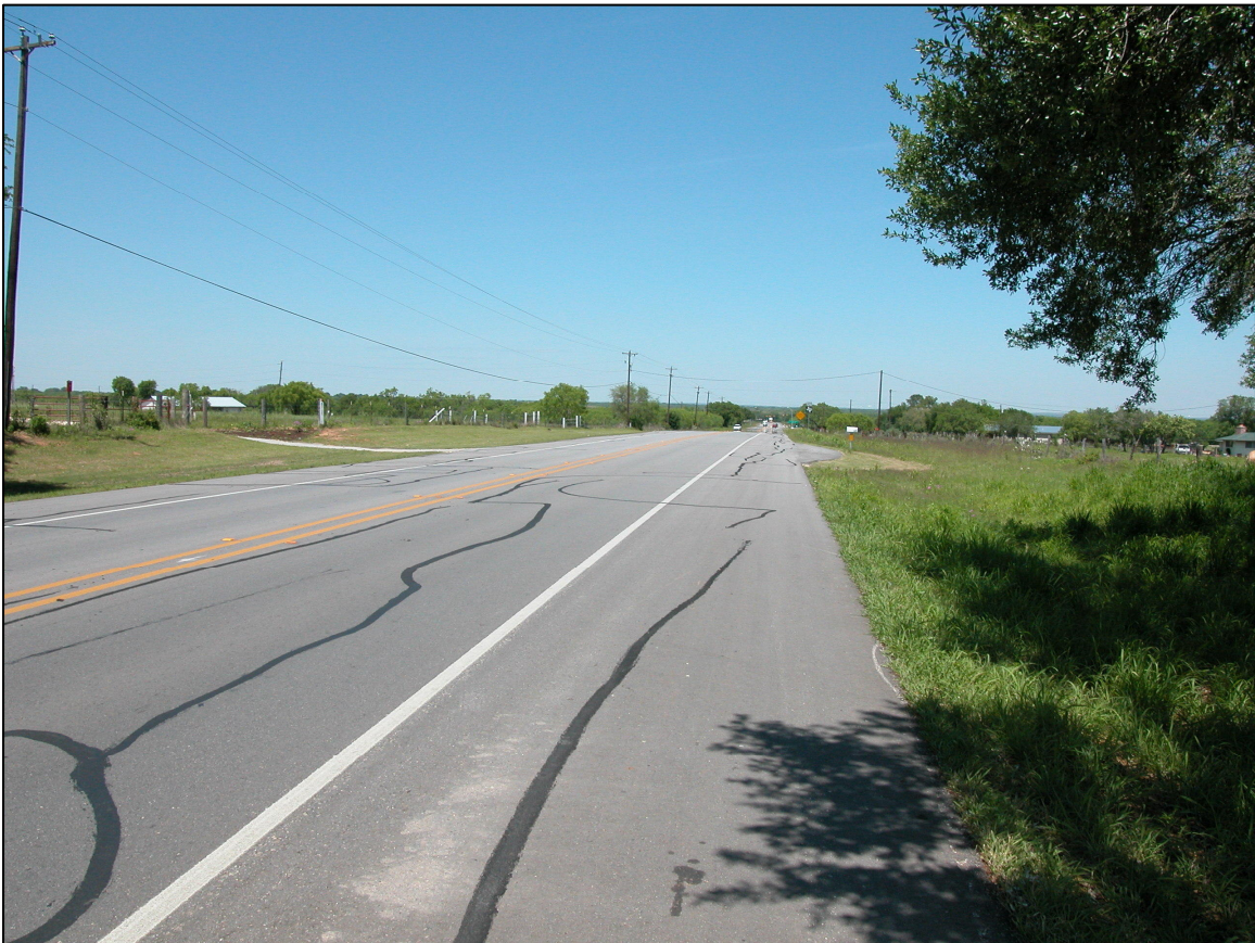
Figure 4.6. SH 16 Test Sites 3 (left lane) and 4 (right lane) on April 13, 2004.
