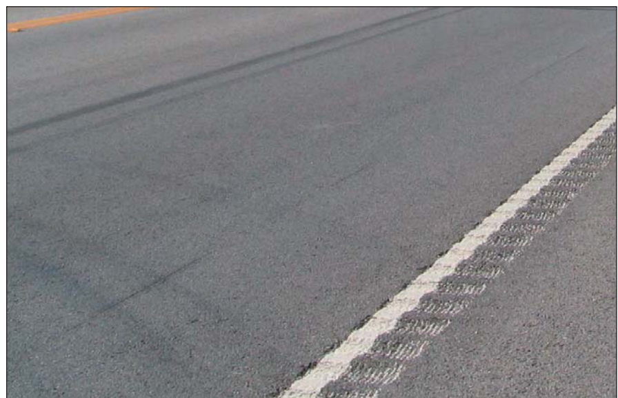
Figure 3. Typical Installation of ERSs.
