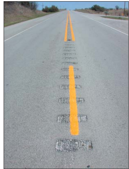
Figure 2. Typical Installation of CRSs.
