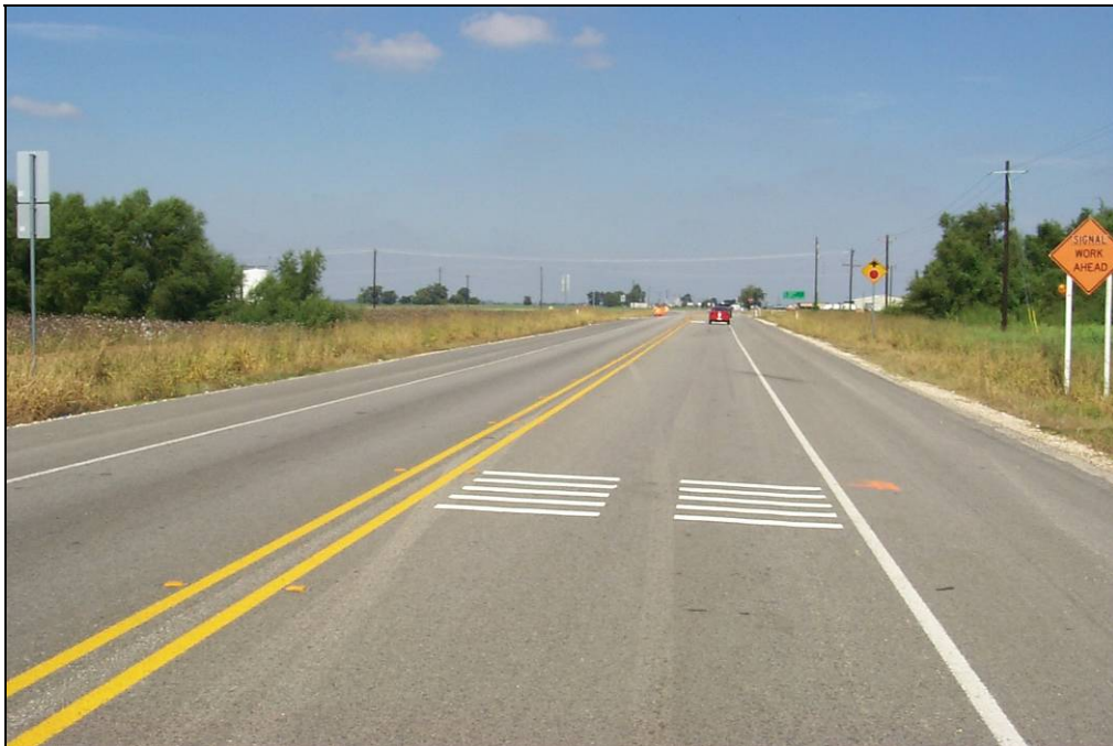
Figure 4. Upstream View of Installed Rumble Strips.
