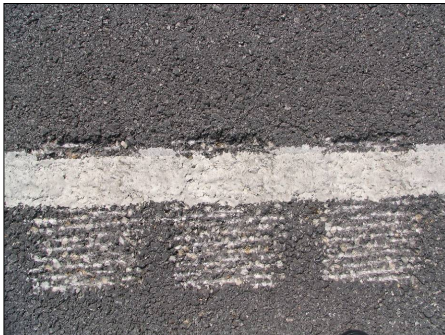
Figure 63. Picture of Edgeline Rumble Strips.
