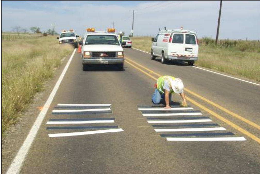
Figure 3. Installation of Rumble Strips.
