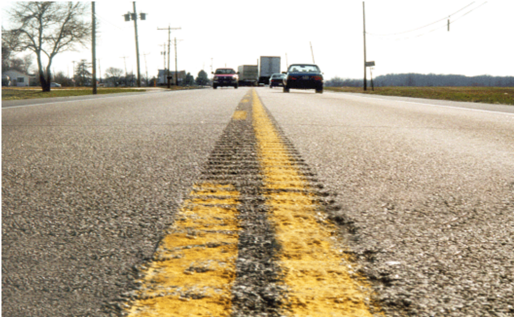
Figure 3. Delaware Centerline Rumble Strips.
