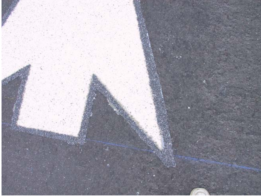
Figure 19. Detail of Completed Contrast Edging.
