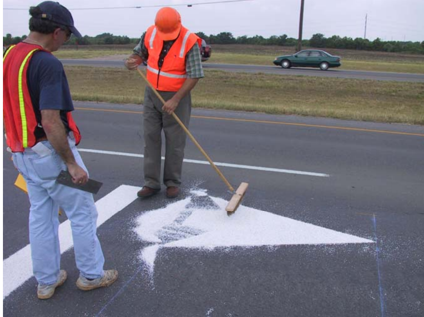
Figure 17. Sweeping Excess Aggregate.
