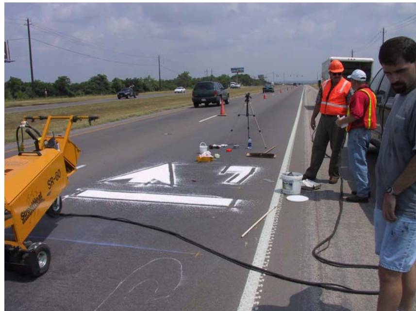
Figure 18. Removing Masking from Symbols.
