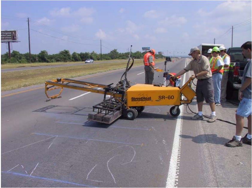
Figure 12. The Streetprint Machine Preheating the Application Area.
