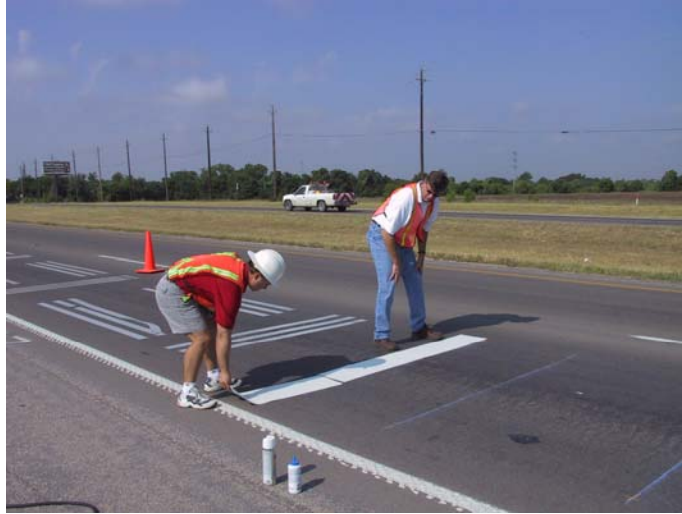
Figure 3. Layout of Preformed Sections before Application.
