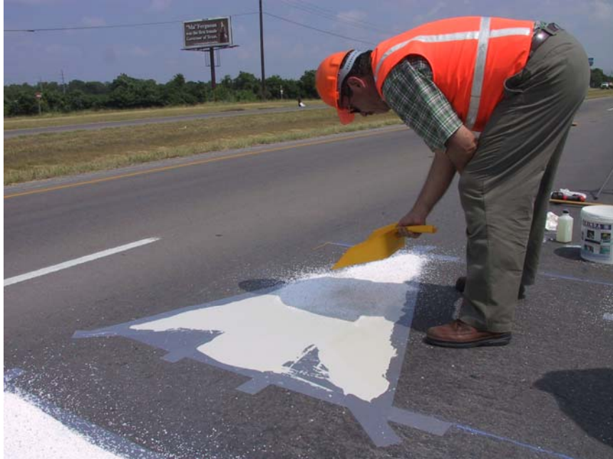
Figure 15. Applying Aggregate to Rocbinda.
