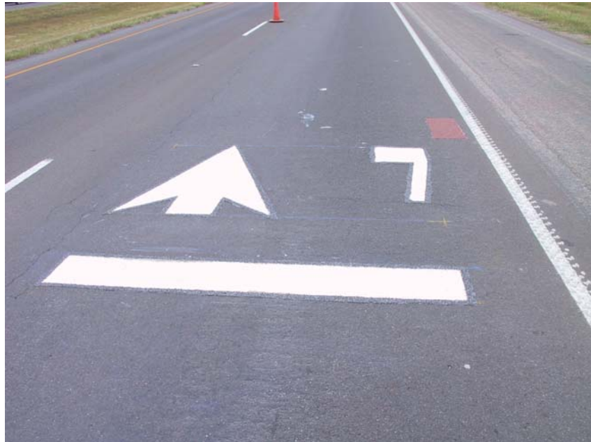
Figure 20. Completed Robinda Segment.
