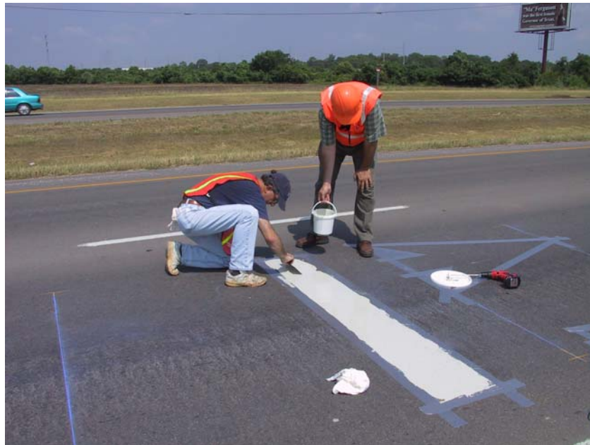
Figure 14. Rocbinda Masking and Binder Application.
