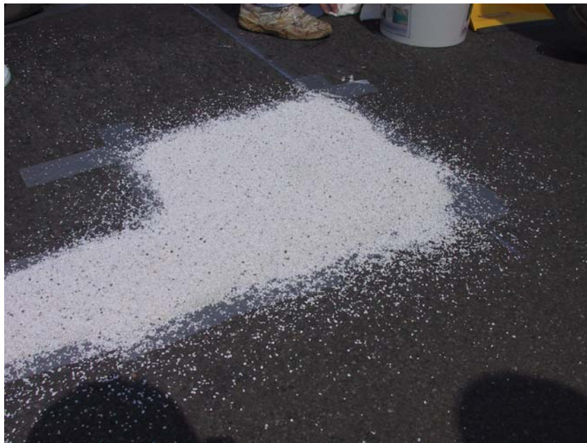
Figure 16. Rocbinda after Aggregate Application.
