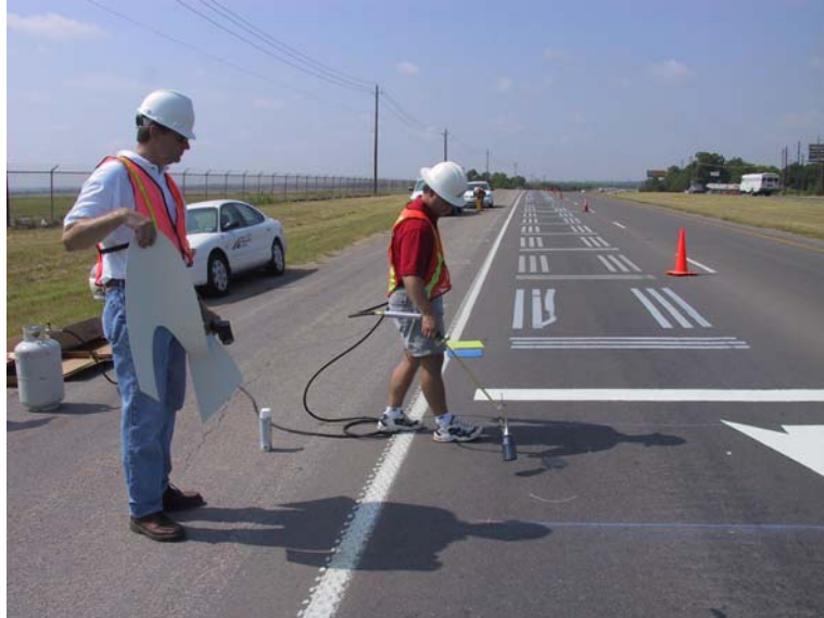
Figure 9. Preheating the Pavement with a Propane Torch.
