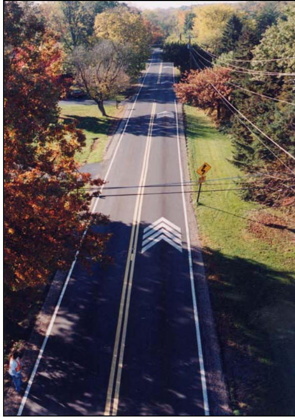
Figure 2. Roadway Marked with Chevron Pattern.
