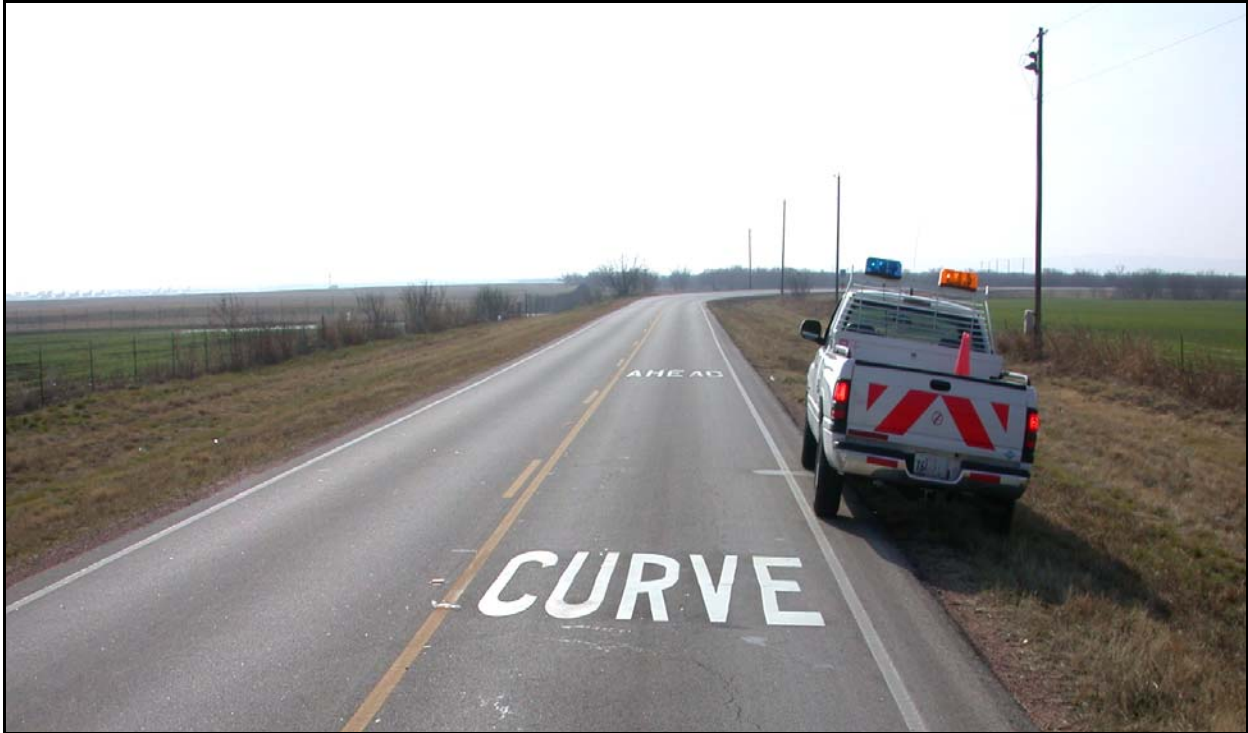
Figure 8. CURVE AHEAD Treatment.
