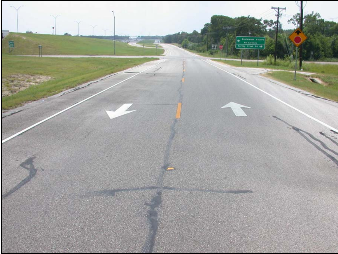
Figure 18. View of Frontage Road Location after Arrow Installation.
