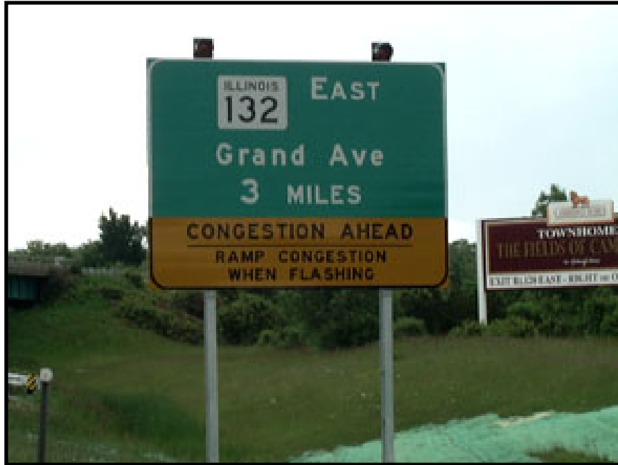
Figure 4-15. Example of Sign Panel on Guide Sign. 1
