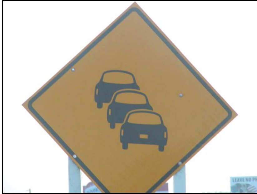
Figure 2-2. Photograph of Pictogram Congestion Warning Sign Used in Field Study.
