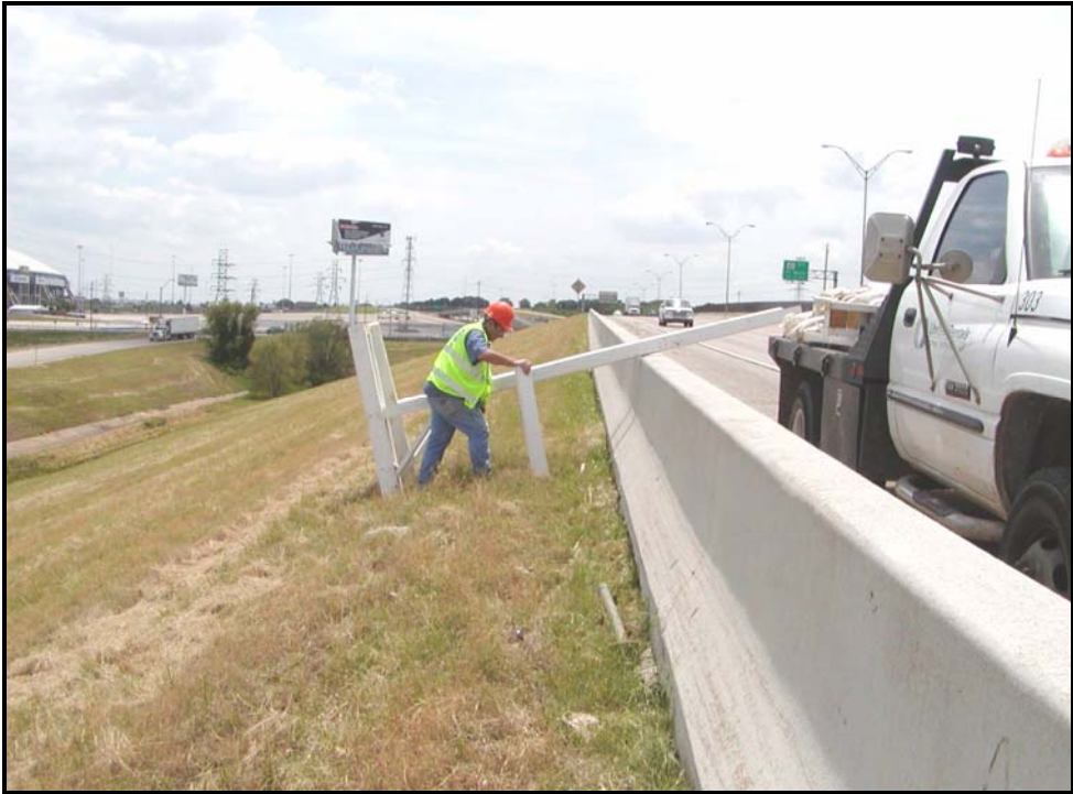
Figure 2-18. United Rental Crews Deploying Signs.
