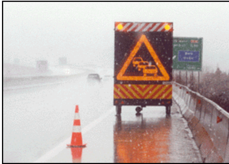
Figure 2-6. Portable Sign Deployment in Turkey. 1
