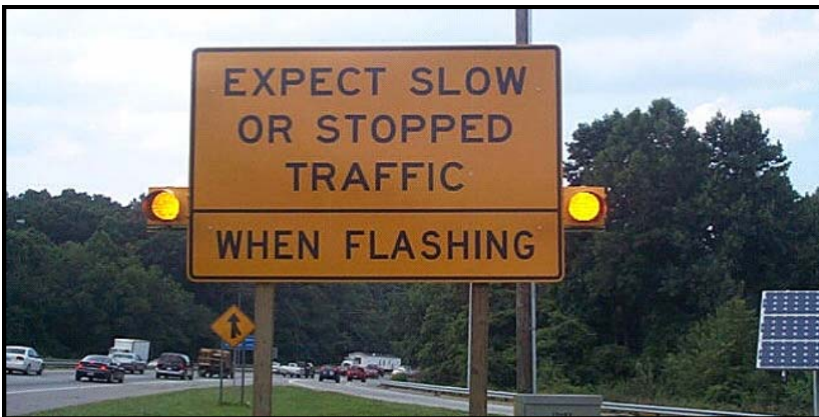
Figure A-1. Picture of Queue Warning Sign on Interstate 26 in Asheville, North Carolina.
