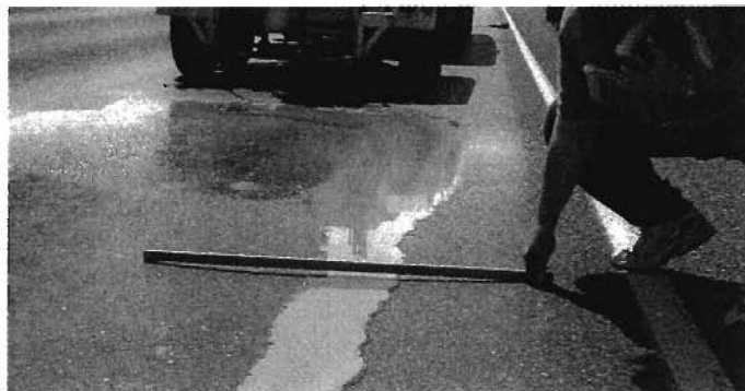
Medium-Severity Rutting
