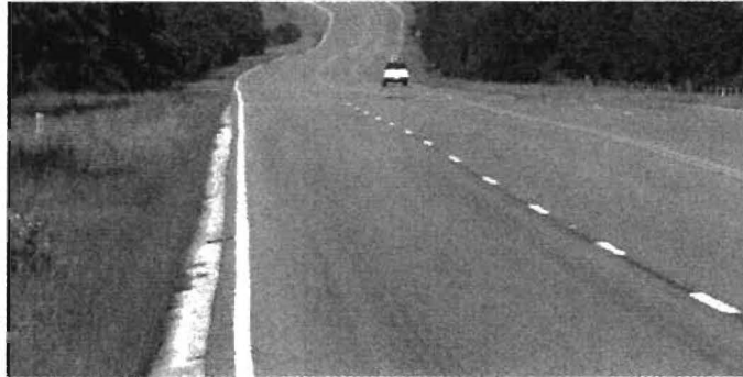
Roughness on Roadway
