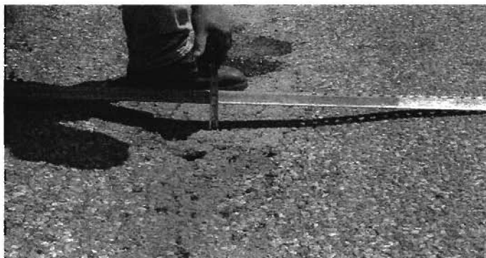
High-Severity Rutting
