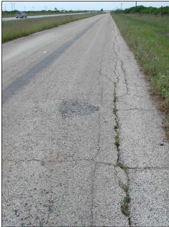
Figure 1.8. I 27 West Side Frontage Road Site 2.
