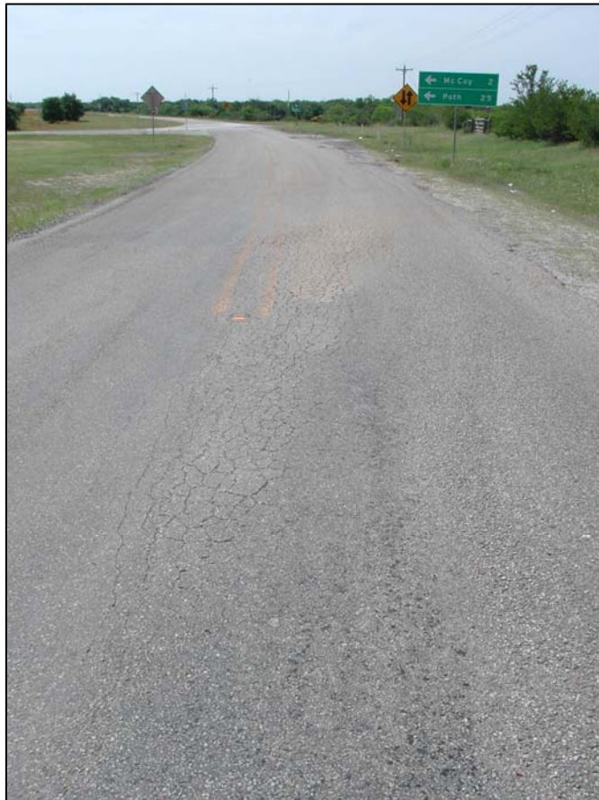
Figure 1.7. I 37 West Side Frontage Road Site 1.
