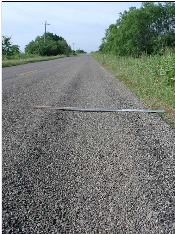
Figure 1.2. FM 1332 WB Toward End of TxDOT Maintenance.
