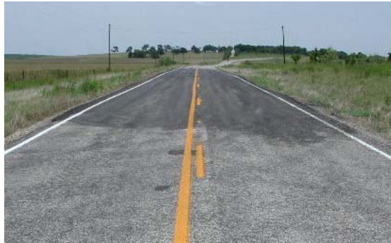
Figure 12. Blade-on Patch on First Geogrid Section on FM 1915.
