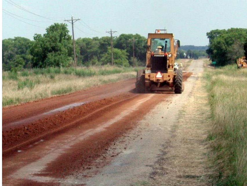
Figure 19. Placement of Recycled Base on FM 2967.
