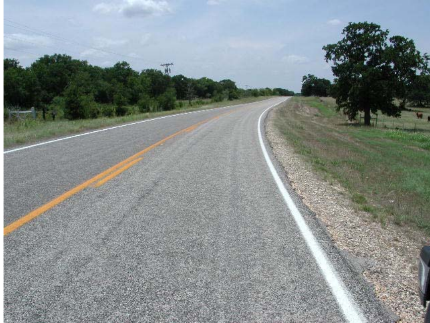
Figure 15. Second Geogrid Section on FM 1915.
