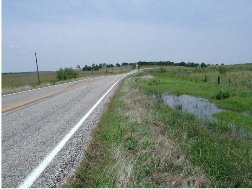
Figure 11. First Geogrid Section on FM 1915.
