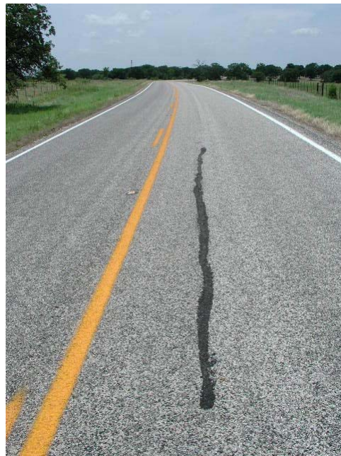
Figure 14. Longitudinal Cracking on Control Section on FM 1915.
