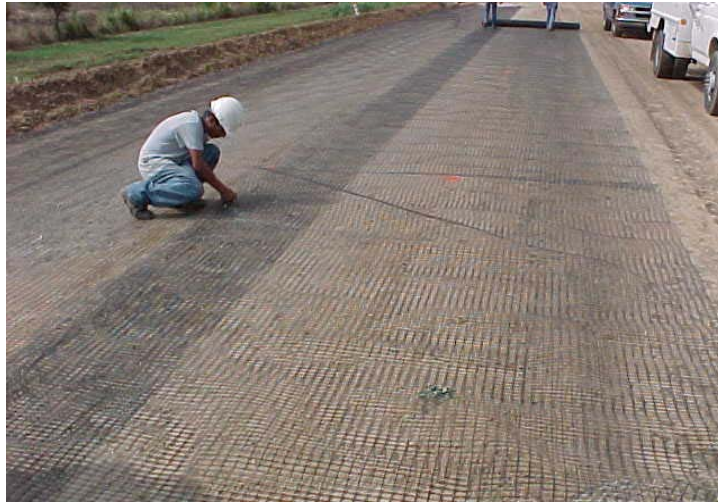
Figure 2. Geogrid Being Placed on Rehabilitation of OSR.
