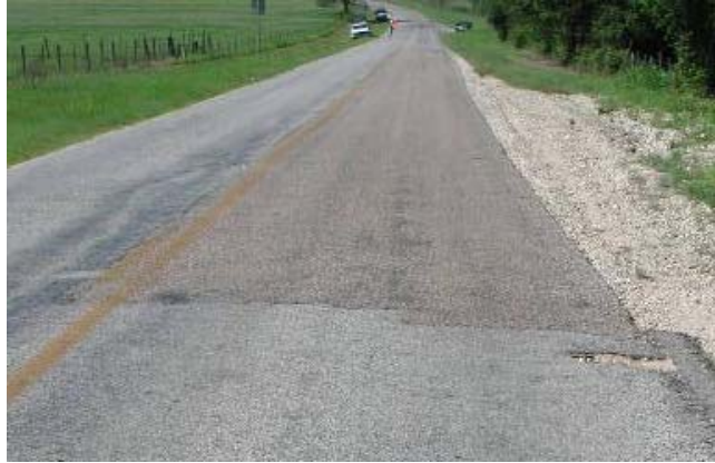
Figure 20. Base Repair Site on FM 20.
