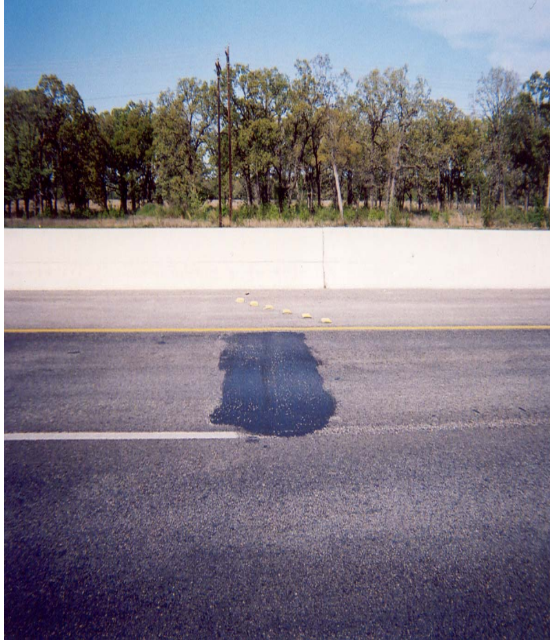
Figure 24. No Paper Joint Used In Underseal Construction.
