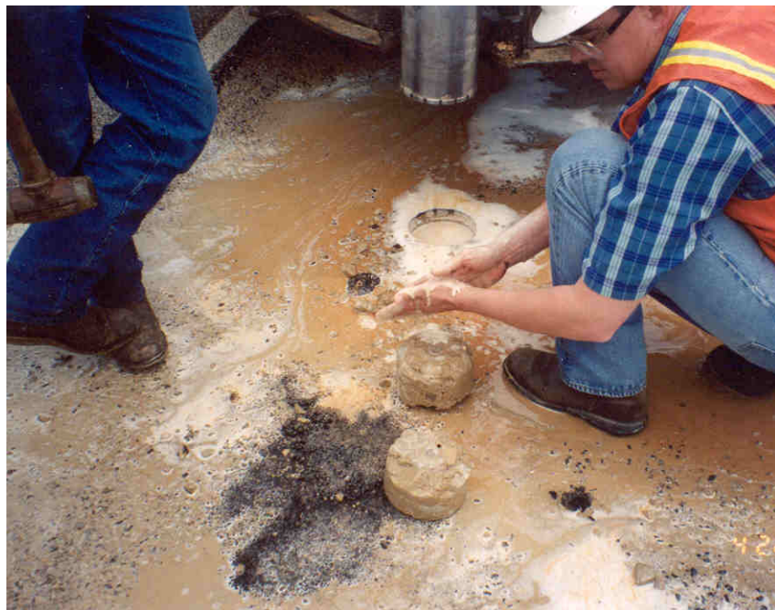
Figure 36. Core of Stabilized Base on Loop 390.
