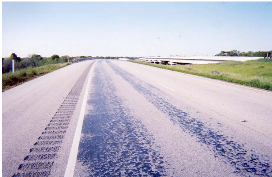
Figure 23. Underseal Flushing on SH 6.
