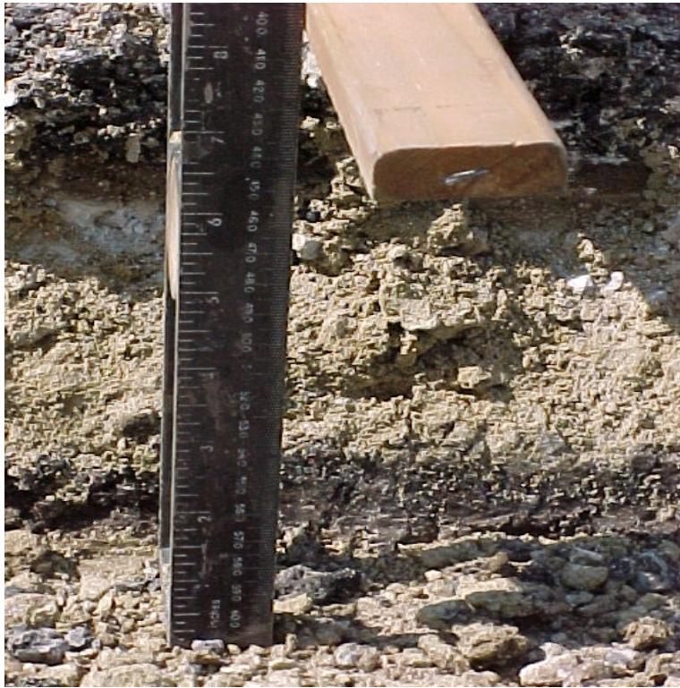
Figure 26. Cross Section of Shoulder Materials.
