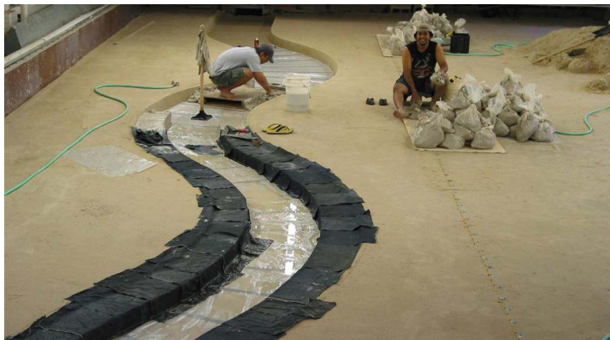
Figure 6.13. Laying the Clay Blocks along the Channel.
