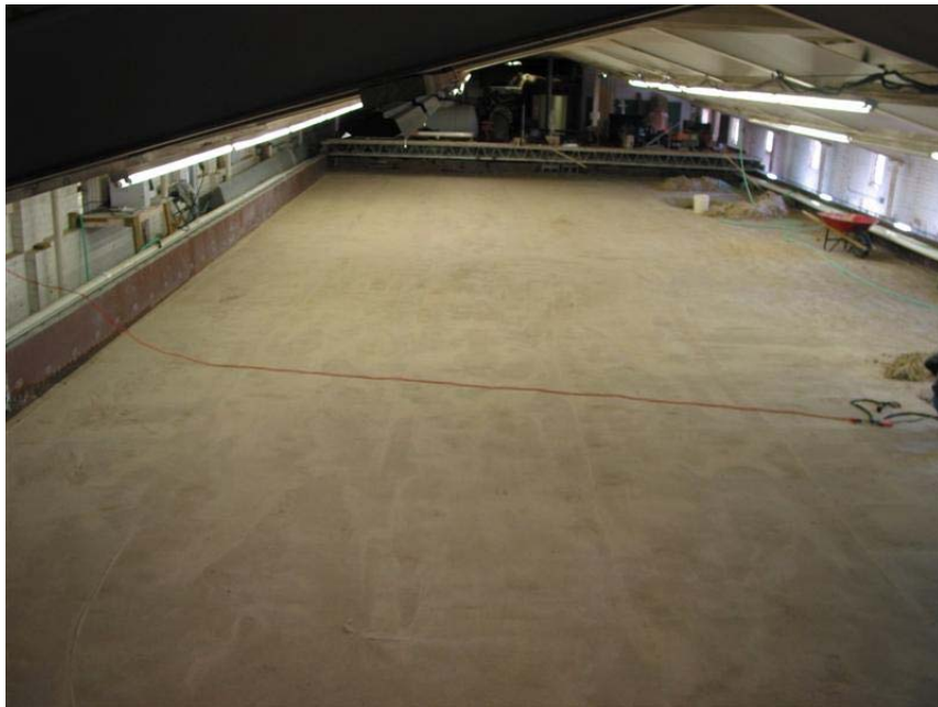
Figure B.4. Completion of Leveling Work.
