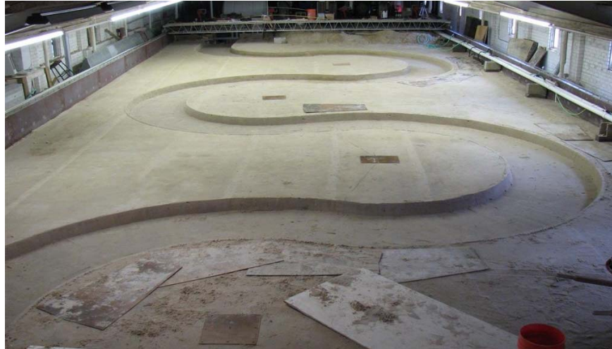
Figure 6.12. Carved Guide Channel in the Sand Bed.
