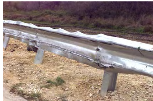
Figure 1-1: Flattened rail
