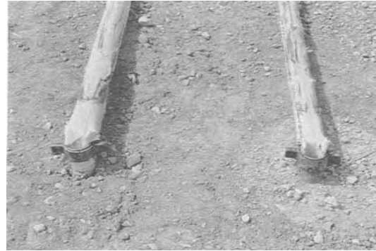
Figure 2-11: Fiberglass post socket system that did not perform as intended
