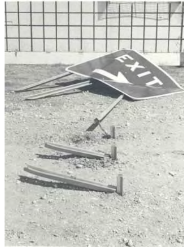
Figure 3-9: U-channel system that performed as intended
