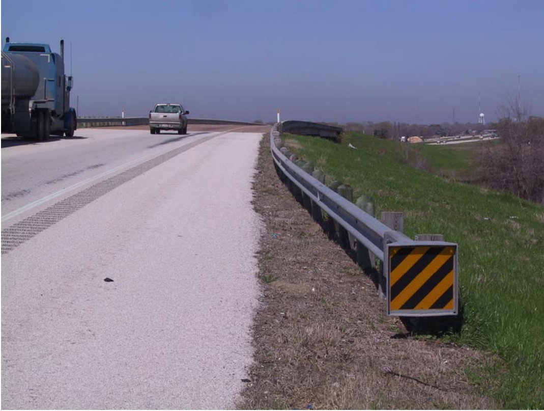
Figure D4: An Example of a Flared ET-2000 Device.
