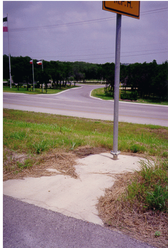
Figure 2-1: Concrete riprap around sign support
