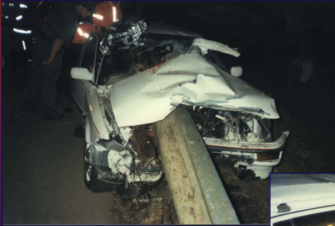
Blunt end of a guardrail (a crash in South Africa where the end-wings are still utilized)
