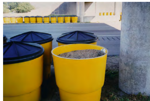
Figure 4-8: Sand barrels should be checked for cracks, loose or missing tops, and loss of sand.
