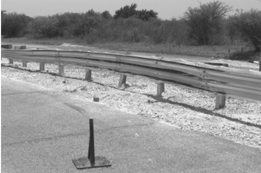
Figure 1-7: Steel post system that performed as intended
