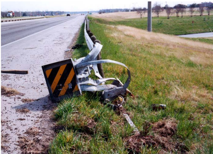
Figure D2: An Example of the Activation of the BEST SGT Device.
