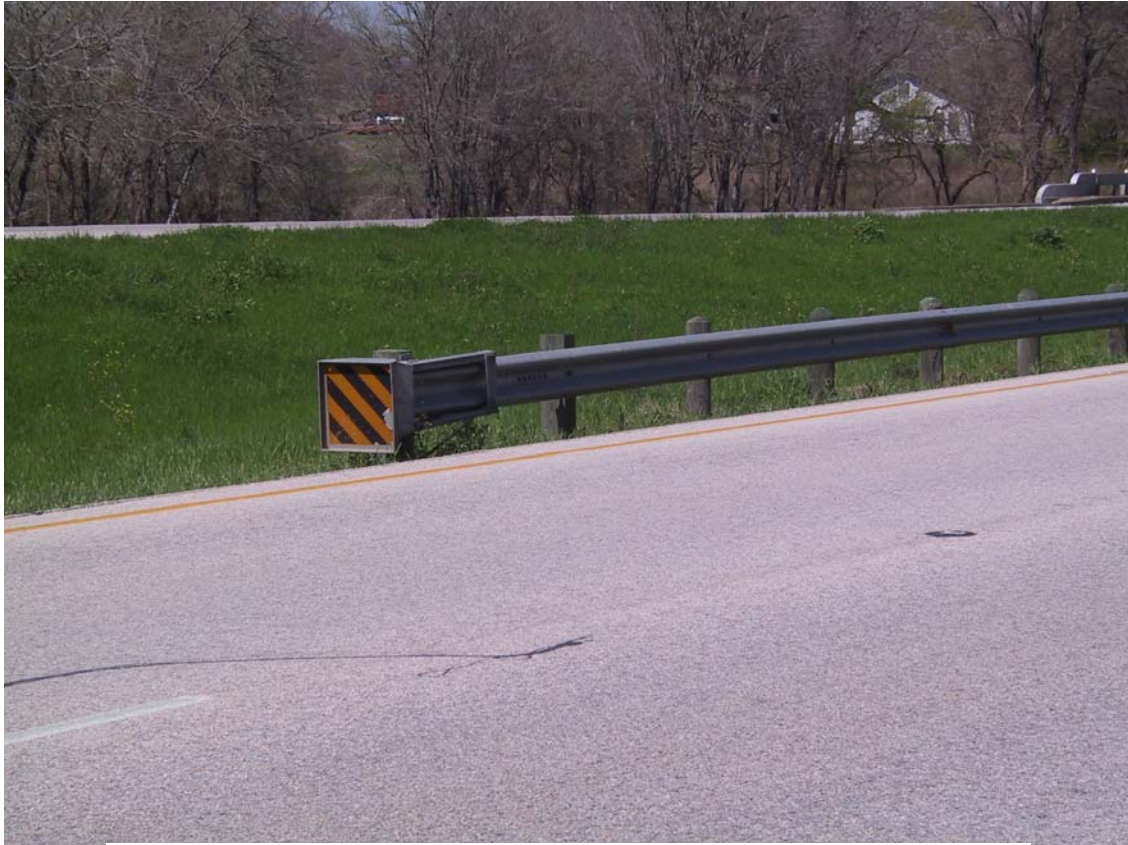
Figure D3: An Example of An ET-2000 Installed On a Slope.
