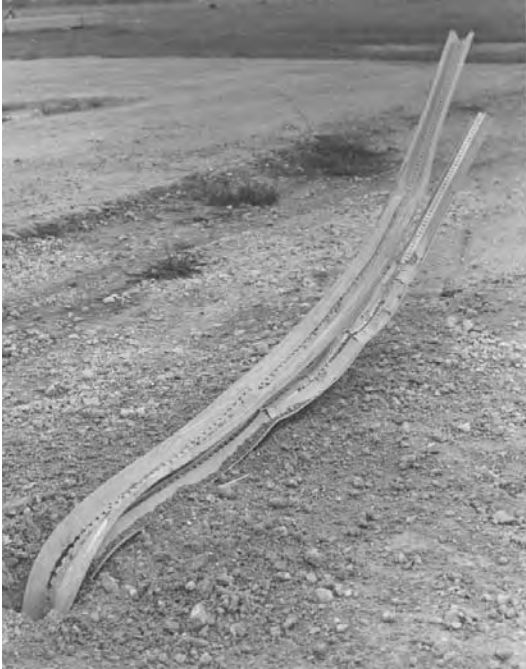
Figure 2-7: U-channel system that did not perform as intended.
