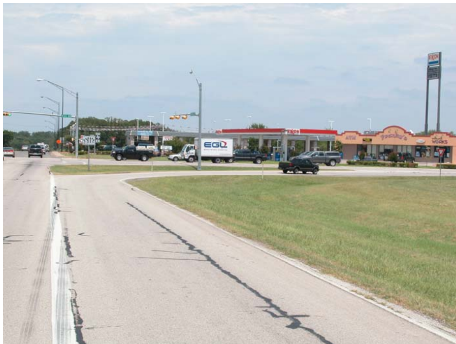
Figure 11. Photograph of Site 2.
