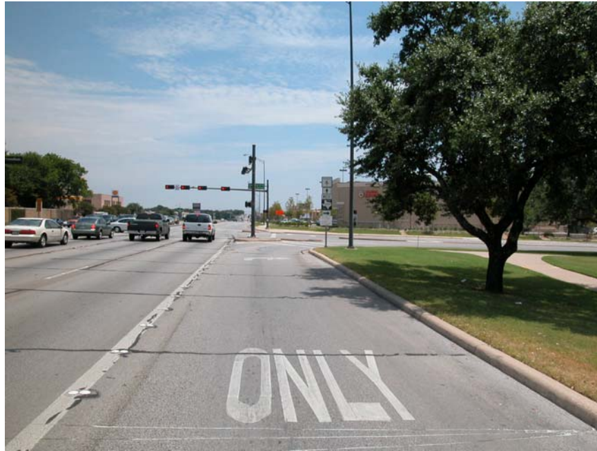
Figure 10. Photograph of Site 1.
